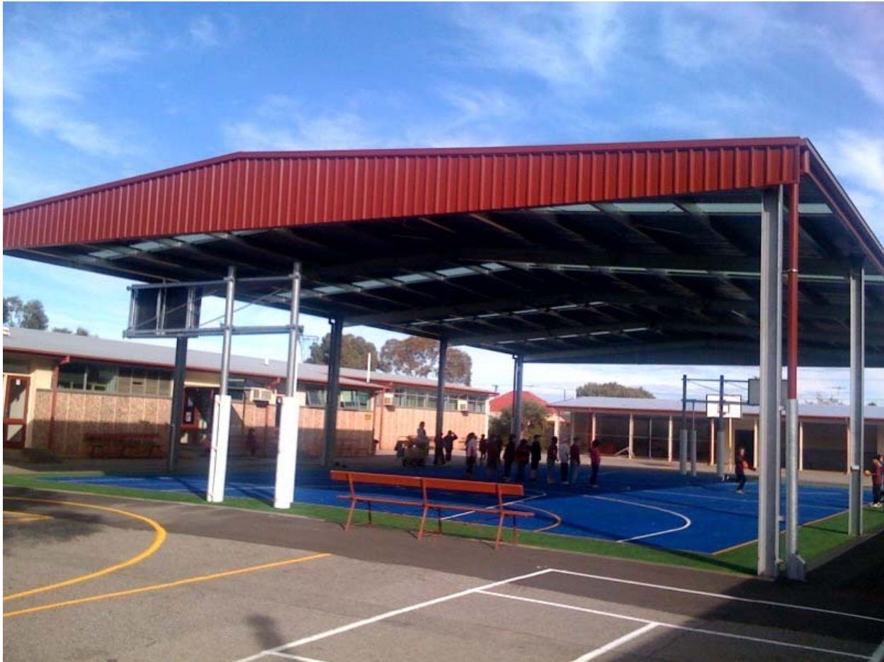
Figure 1. This COLA is located at Murray Bridge South Primary School and was completed in May 2010
