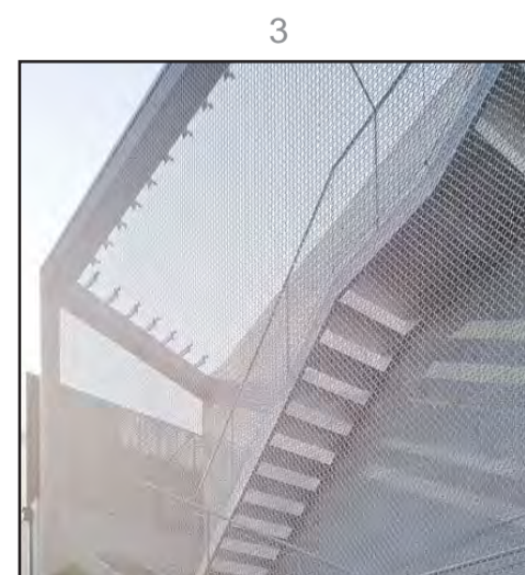
3 ARCHITECTURAL METAL MESH FACADE
