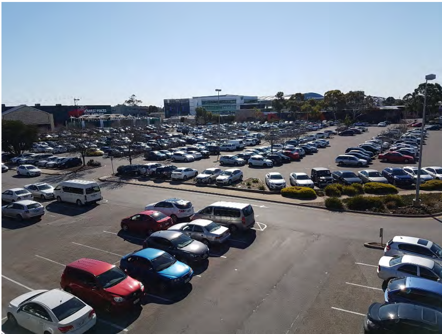
Photo 1 – Existing northern car parking area (looking north)
