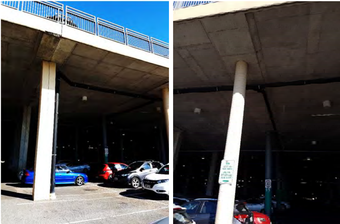
Photo 4 – Example of roof car park drainage system
