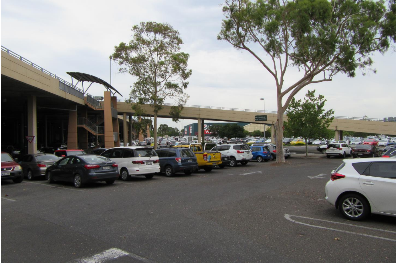
Image 7 – Existing car park and ramp looking west.
