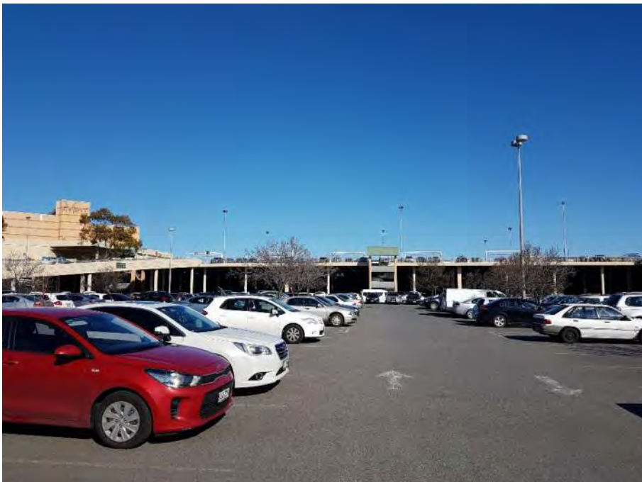
Photo 3 – Undercover and roof car parking area (looking south)
