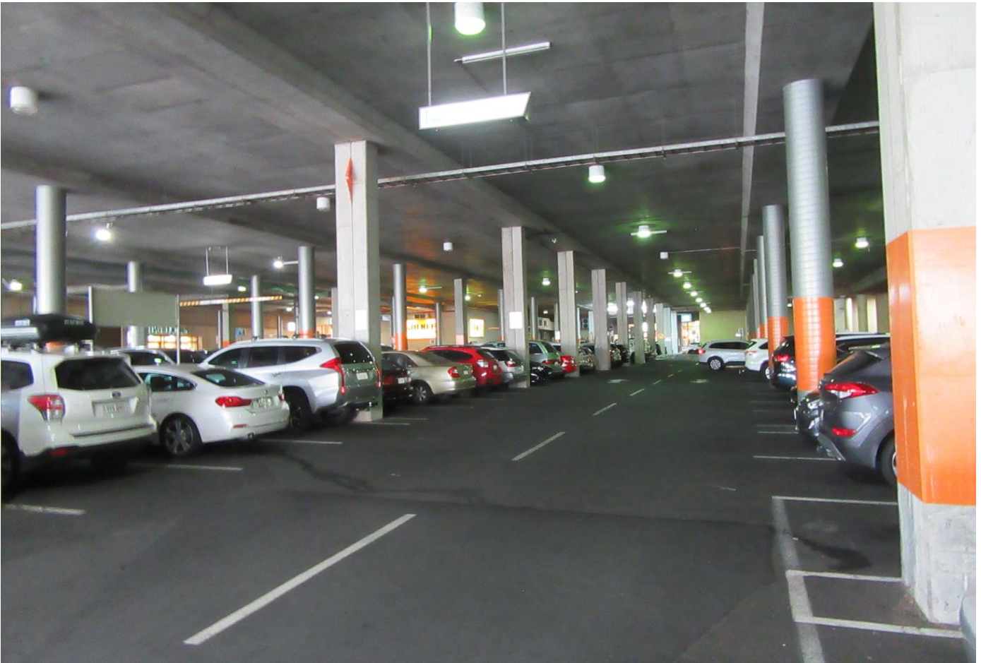
Image 4 – Under-croft car park looking south to south-east
