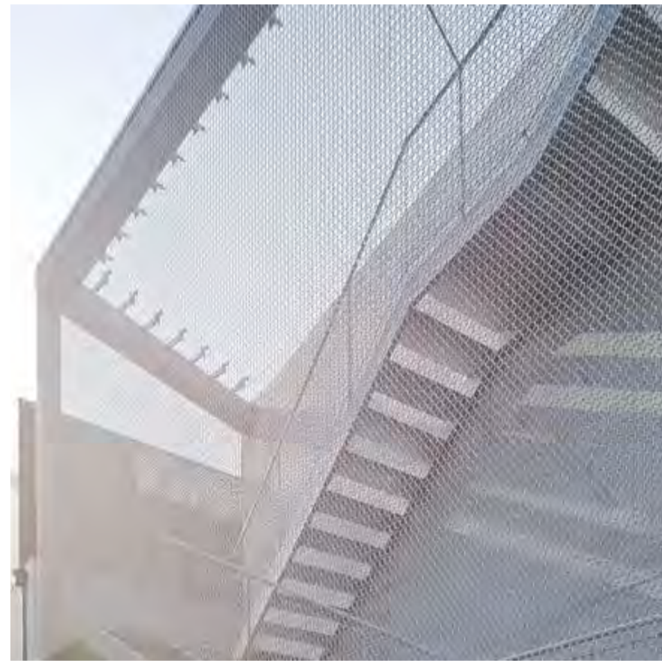
ARCHITECTURAL METAL MESH FACADE
