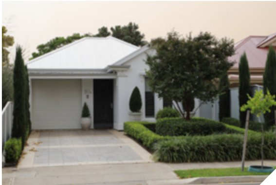
Example of minor infill created by a demolition and resubdivision
