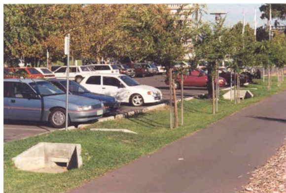
Grassed swale drain. Hackney Road
