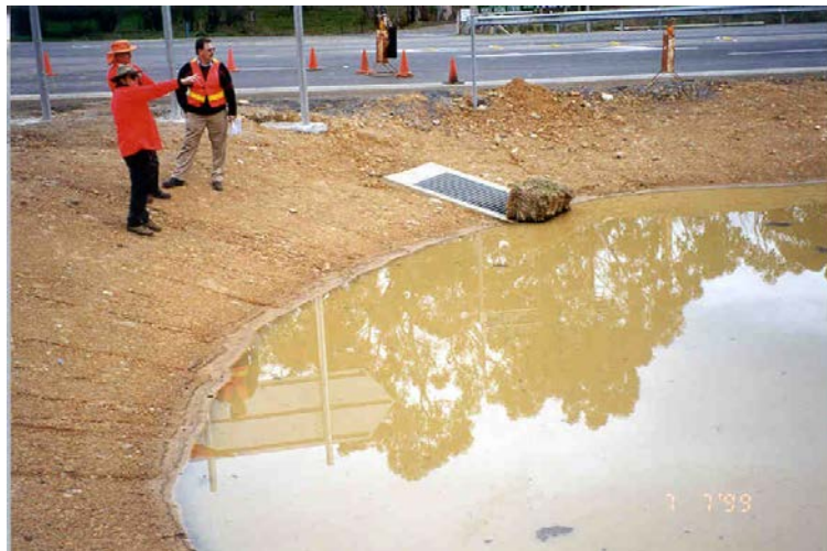
Wet detention basin. Chain of Ponds
