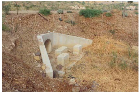
Concrete energy dissipater. Southern Expressway
