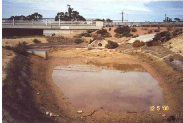
Dry Detention Basin. Blanchetown Bridge
