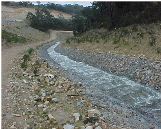
Gabion stabilised drainage line.
