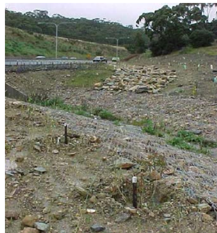
Rock and gabion stabilisation.
