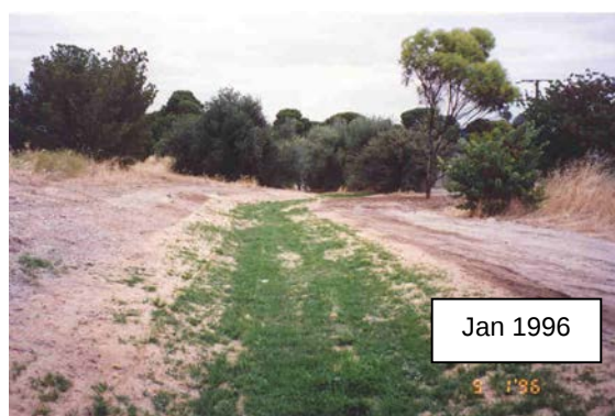
Vegetative stabilisation measures – matting and grasses Panatalinga Road/Railway Terrace, Reynella
