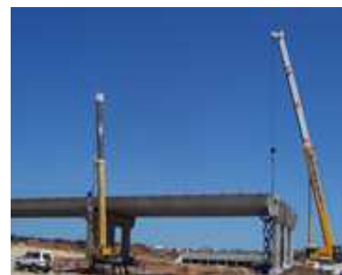
Pictures above: Example of bridge works, erection method of Super T beams. Photographs provided by Bardavcol.
