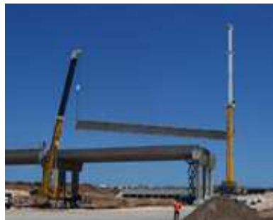
Pictures above: Example of bridge works, erection method of Super T beams. Photographs provided by Bardavcol.
