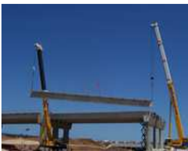
Pictures above: Example of bridge works, erection method of Super T beams. Photographs provided by Bardavcol.
