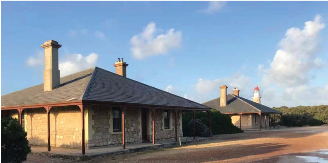
Figure 2.2 Existing State Heritage listed Cape du Couedic Lighthouse Keepers' Cottages with Lighthouse in the background
