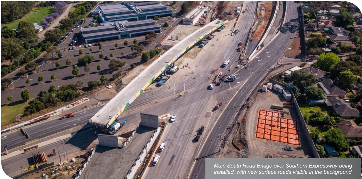
Main South Road Bridge over Southern Expressway being installed, with new surface roads visible in the background
