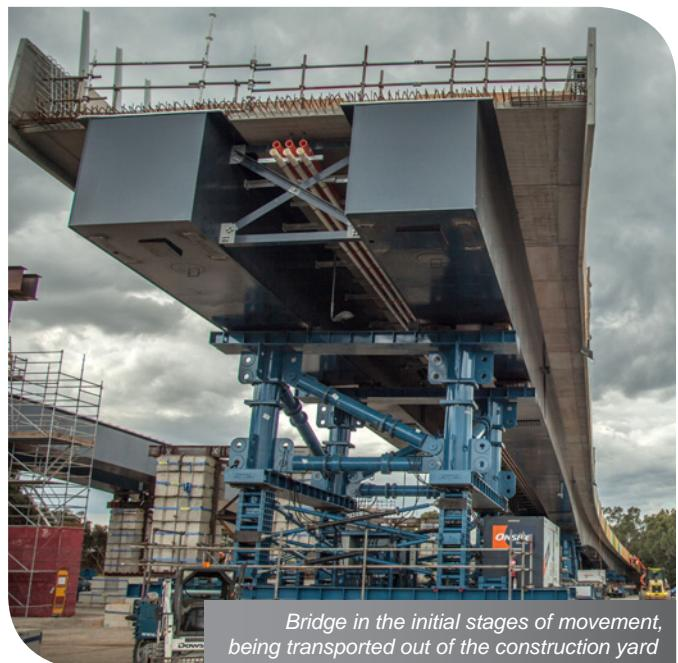
*Bridge in the initial stages of movement, being transported out of the construction yard*
