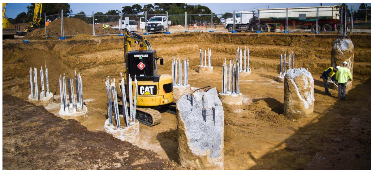
Group of 12 piles and excavation for the pile cap
