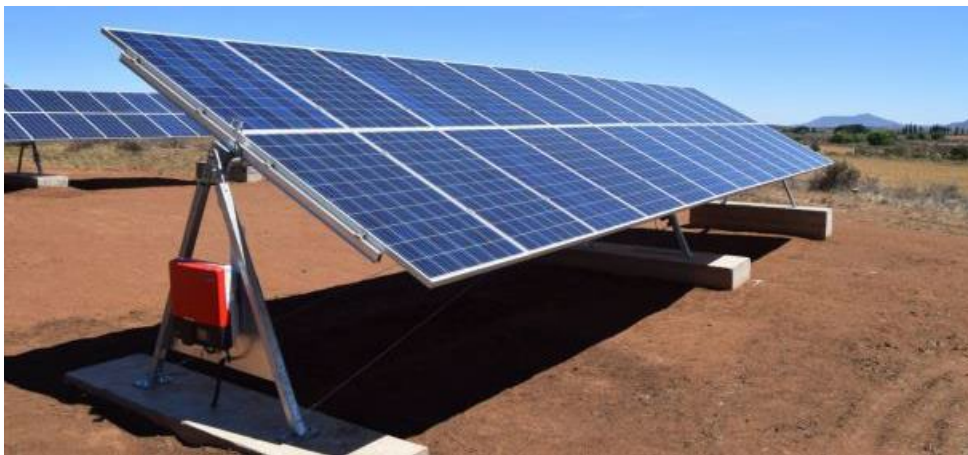
Figure 16 Single Axis Solar PV Array mounted on a concrete ballast (note: Mannum will likely be piles)
