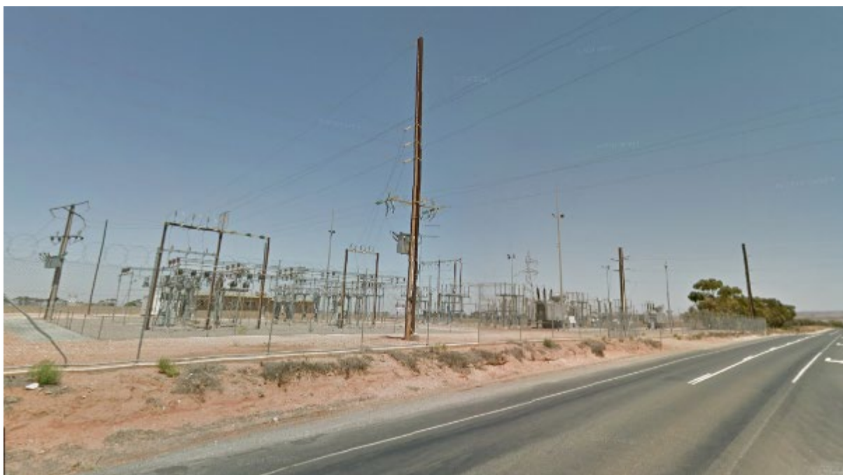
Figure 17 Mannum SAPN and ElectraNet Substation
