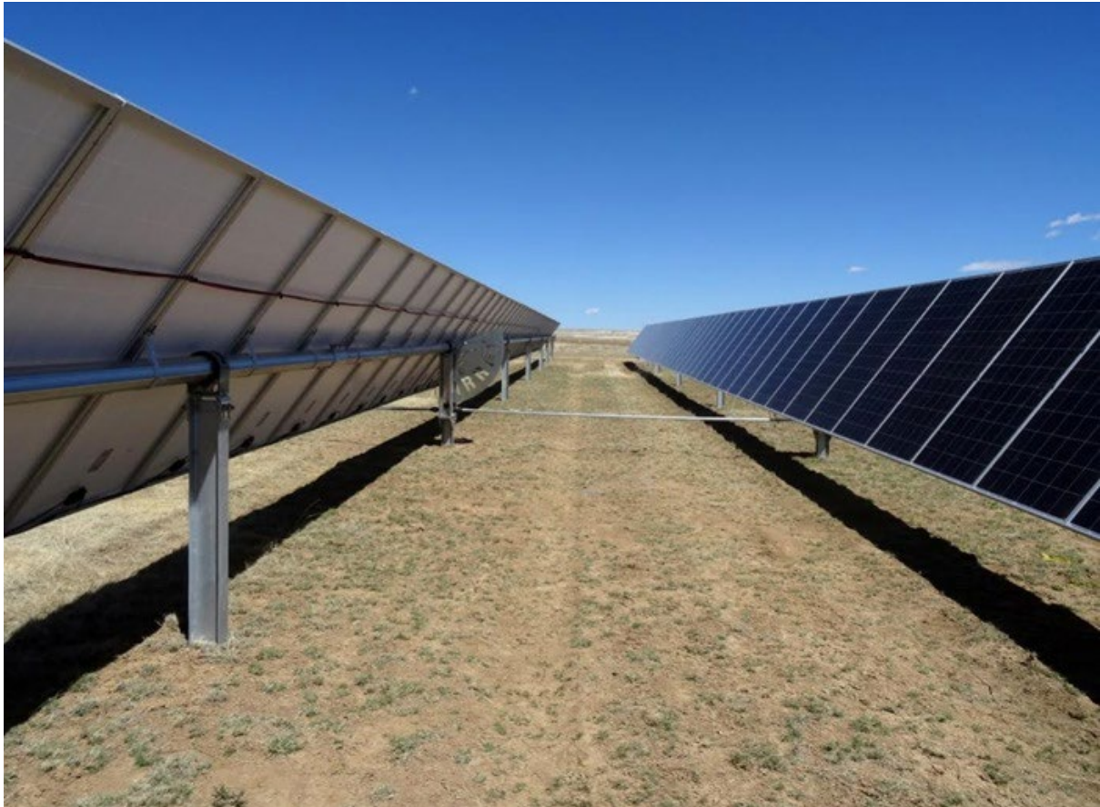
Figure 2 Example Single-axis Tracking Solar PV Array – pile mounted
