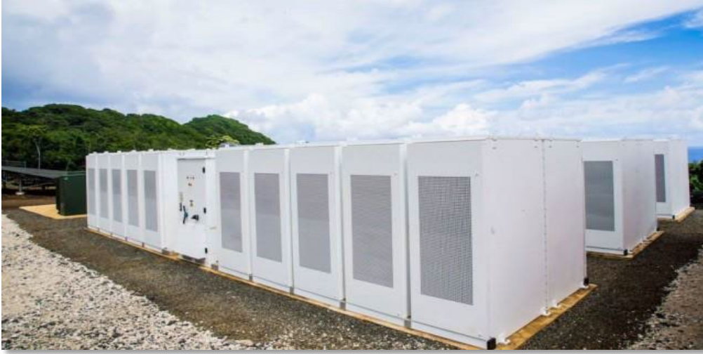
Figure 18 Example Battery Storage System
