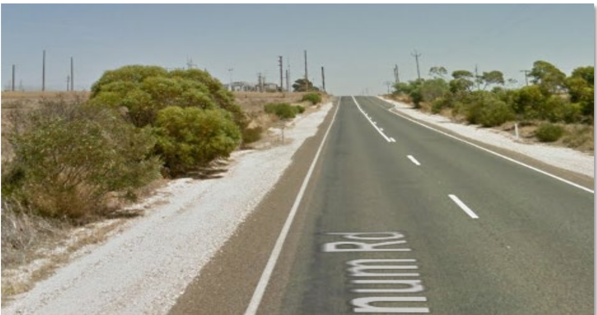
Figure 21 Location of approved site access for stage 1 from Mannum Road (150m south of Fig.19)
