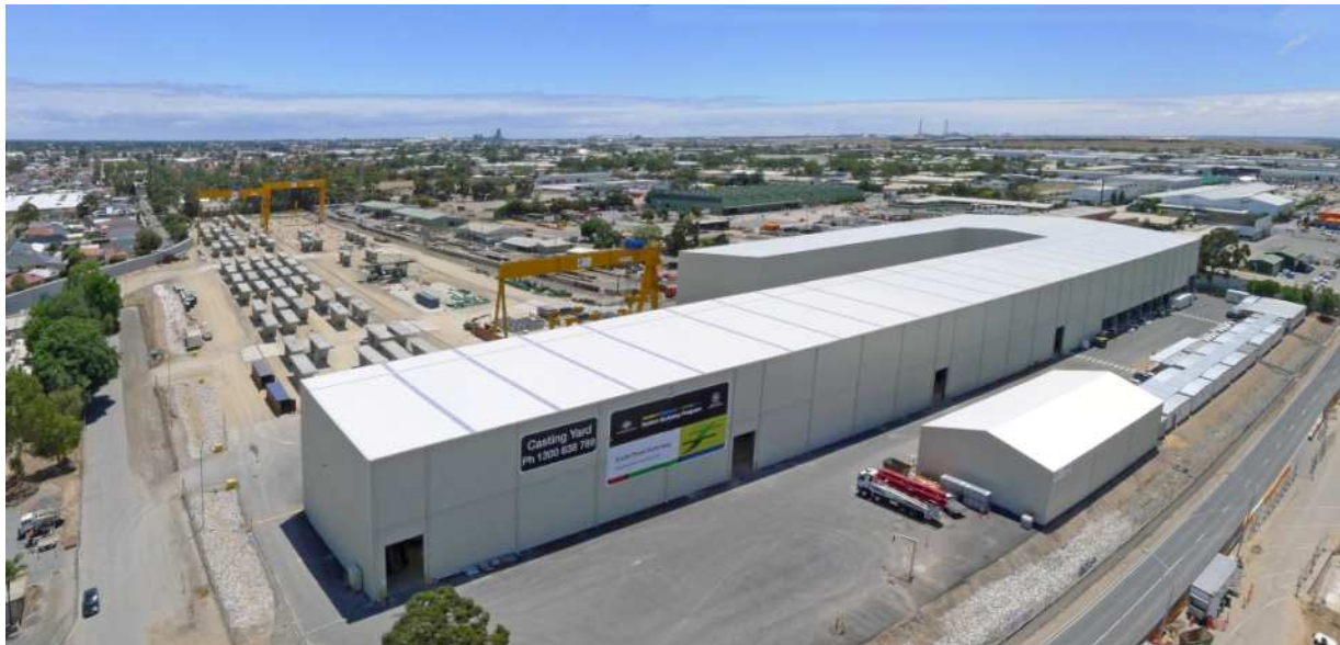
Casting Yard and shed at 628-638 South Road Angle Park
