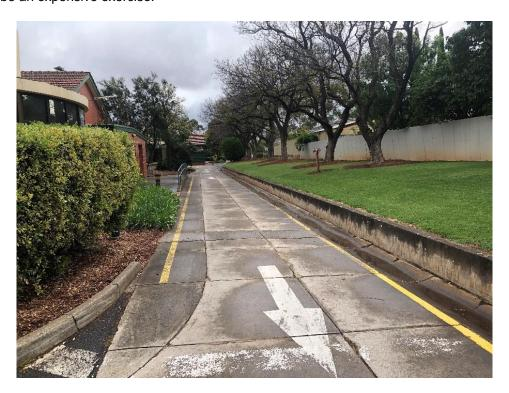
Figure 7n - Possible Road Widening is Likely to be Expensive Due to the Existing Retaining Wall (East End of Building)
