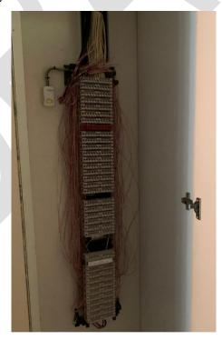
Figure 20. Building 71 & 72 (Ward 1 + 2) main communication building distributor (TC-17)
