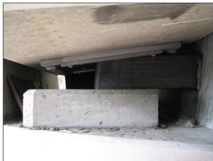
Figure 8 Typical Bearing Movement: Pier 3
