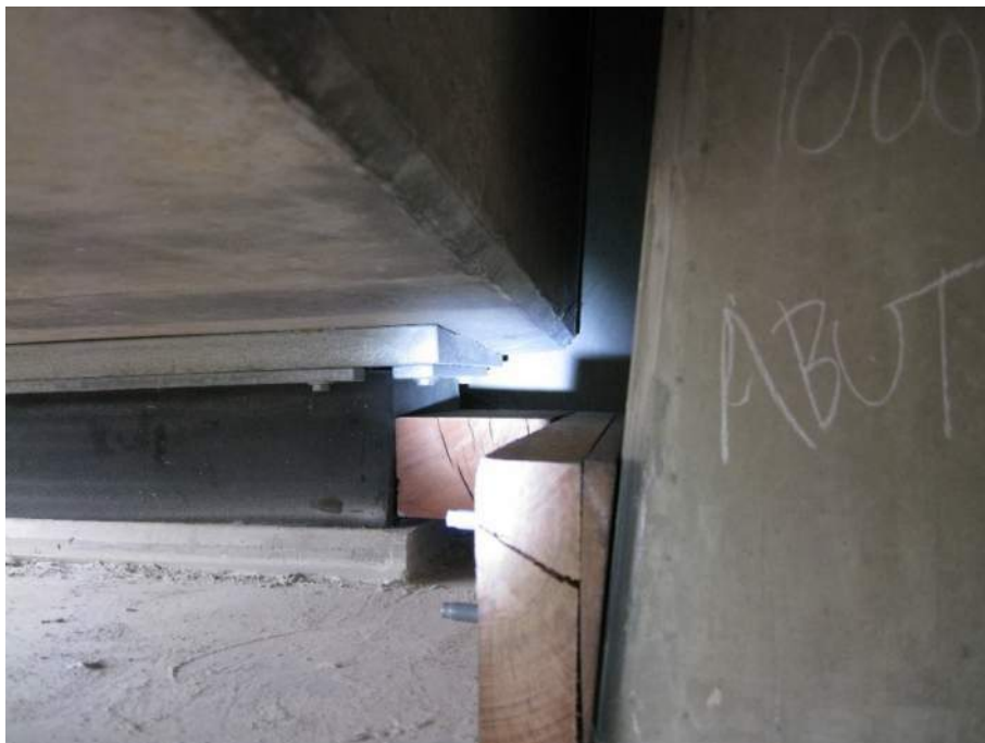
Abutment A Bearing Rotation
