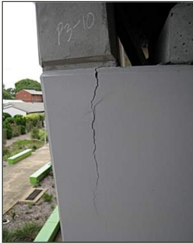
Figure 14 Cracking to pier headstocks
