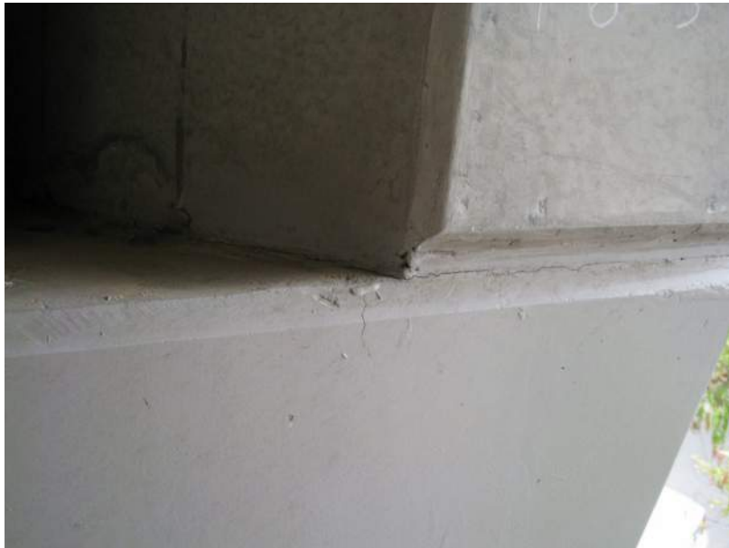
P6 East Wall Cracking
