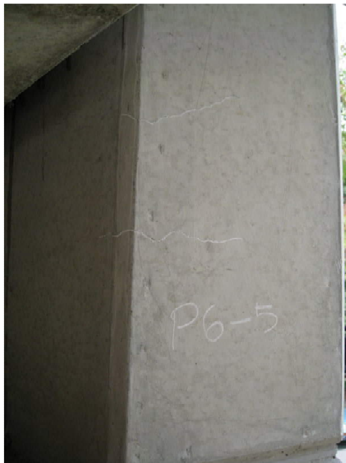
P6 East Wall Cracking
