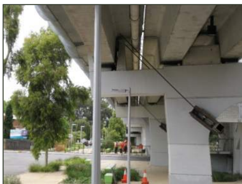
Figure 1 Temporary stabilising tiebacks
