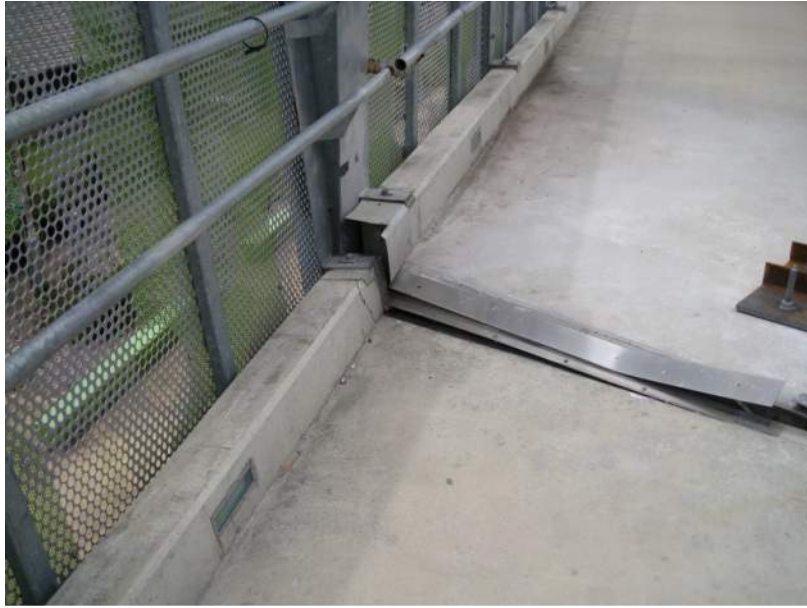
Joint Damage Typical
