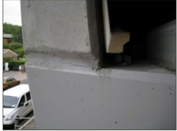
Figure 11 Cracking at keeper wall
