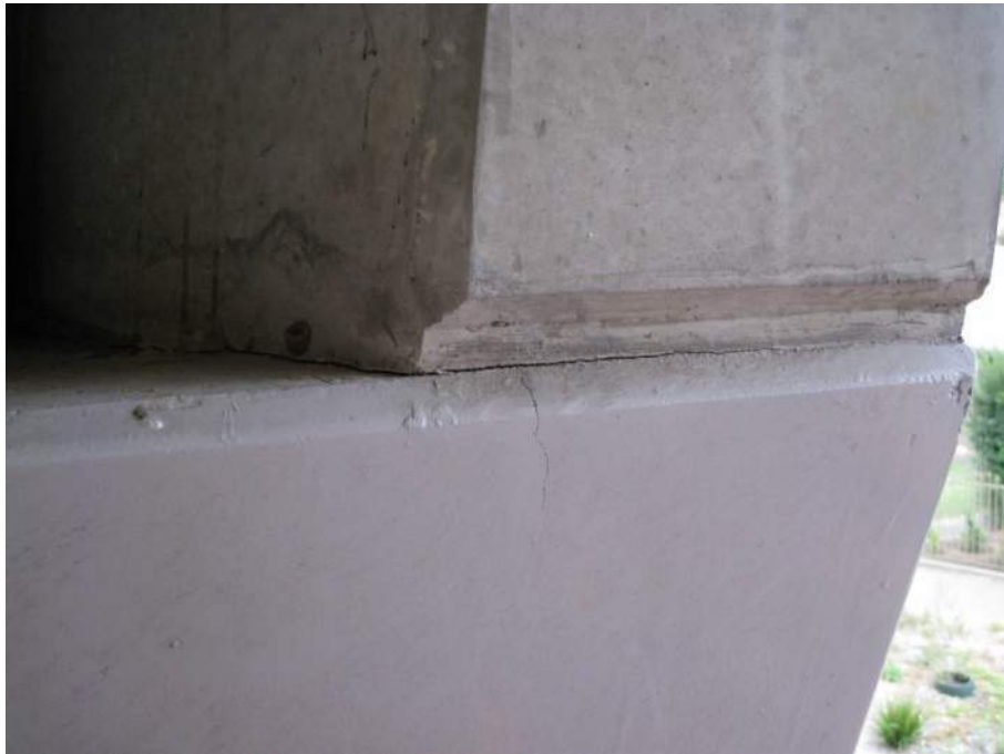
P2 East Wall Cracking
