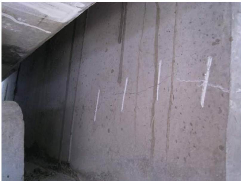
P5 East Wall Crack inside Face
