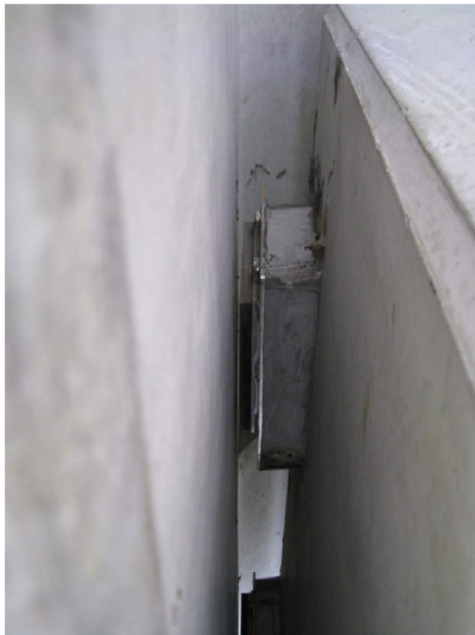
P7 West Side Bearing Separation
