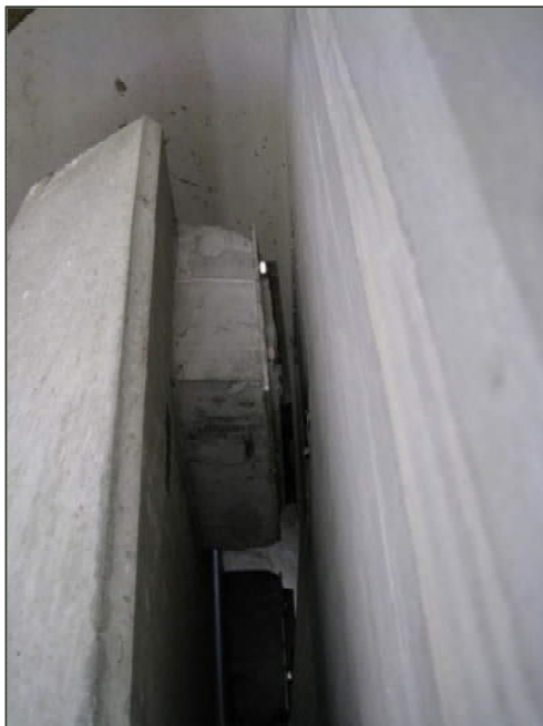
Figure 13 Side bearing separation
