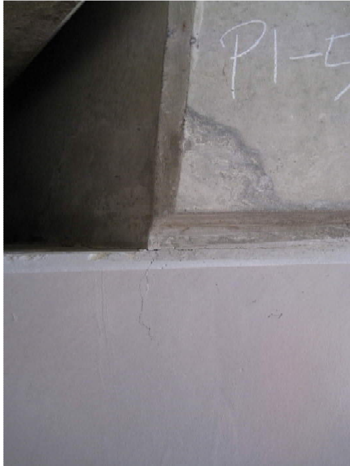
P1 East Wall Cracking
