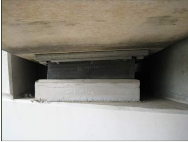
Figure 12 Girder rotation and bearing movement evident
