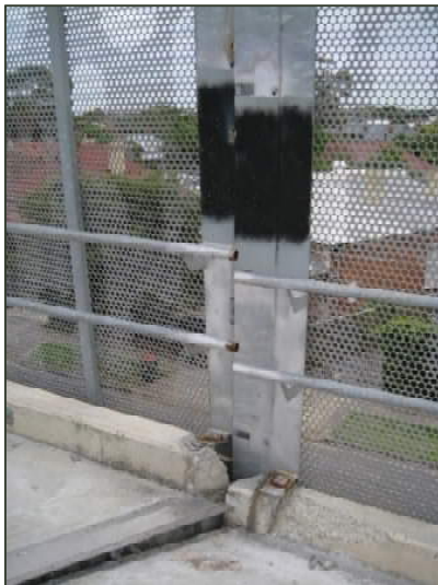
Figure 16 Handrail misalignment
