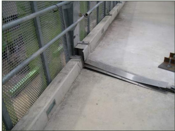
Figure 17 Deck joint damage
