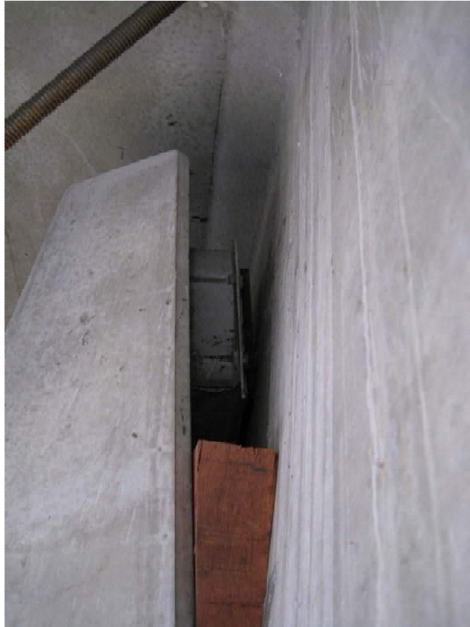
P4 East Side Bearing Separation
