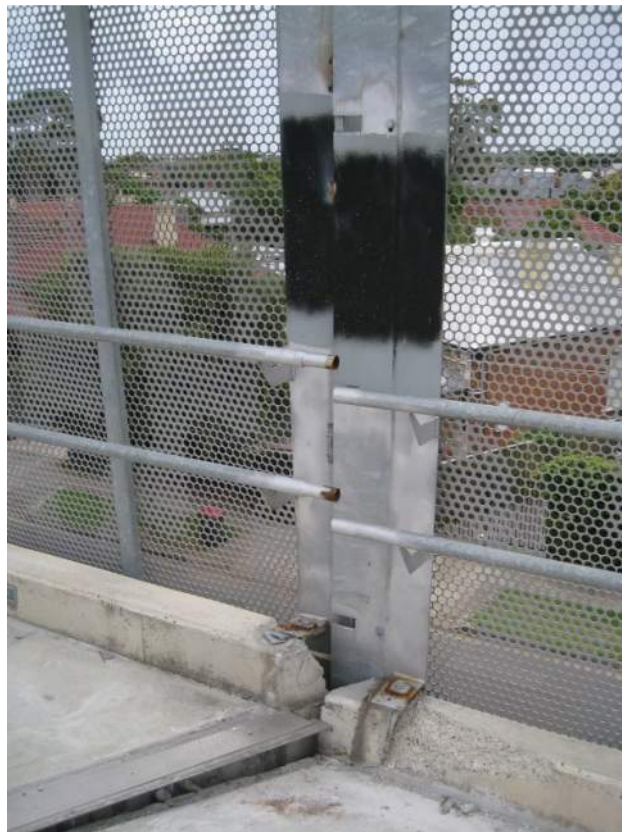
Handrail Misalignment
