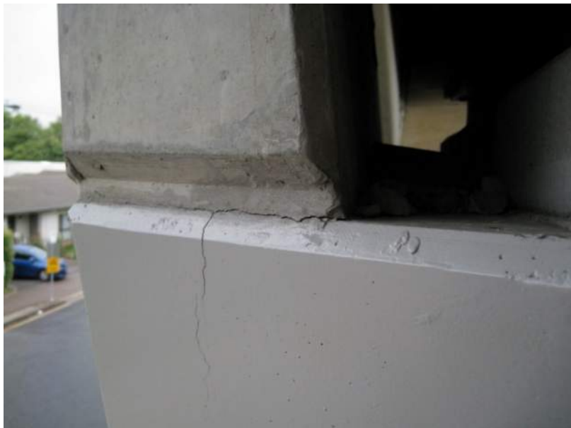
P2 West Wall Cracking
