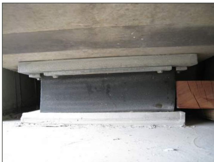
Figure 10 Bearing at Abutment A
