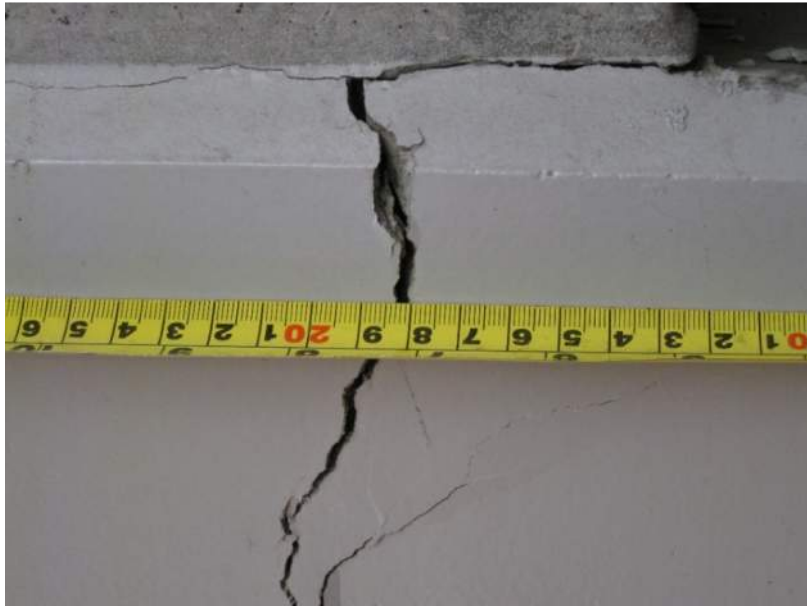
P3 West Wall Cracking
