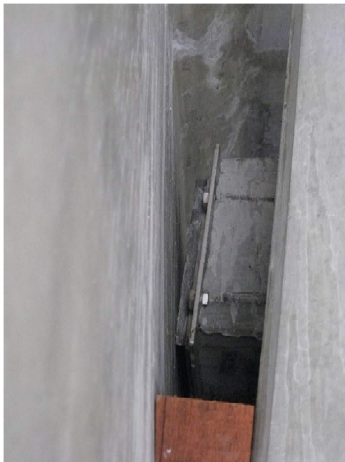
P4 West Side Bearing Separation
