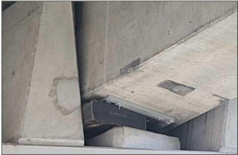
Figure 15 Girder dislodgement due to excessive bearing movement
