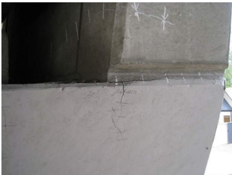
P4 East Wall Cracking
