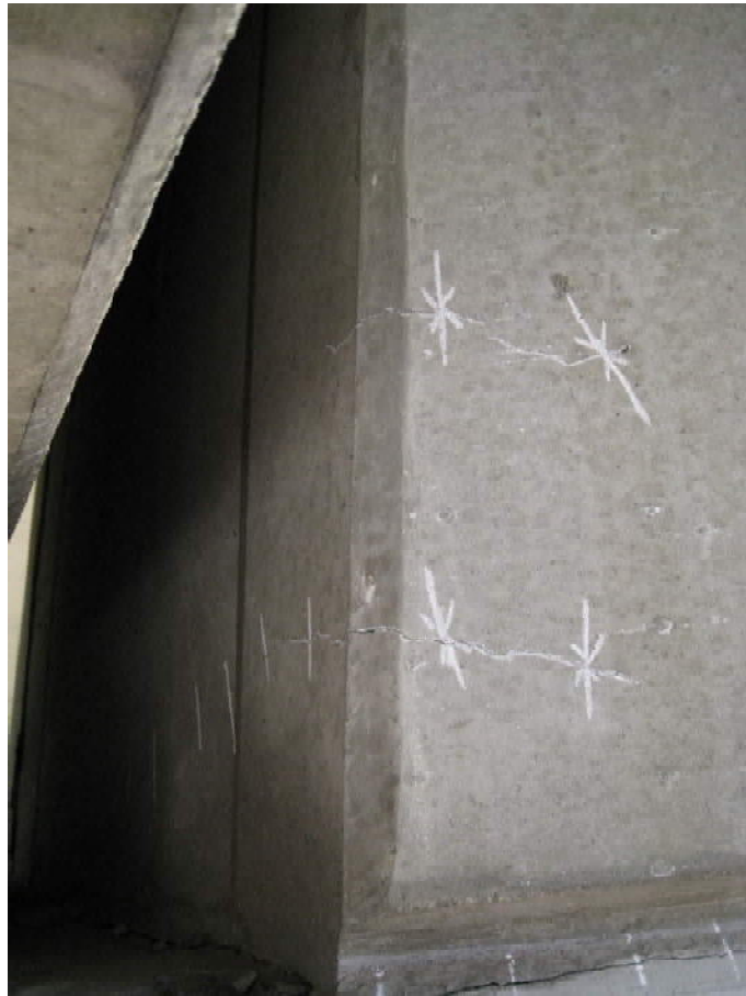
P4 East Wall Cracking
