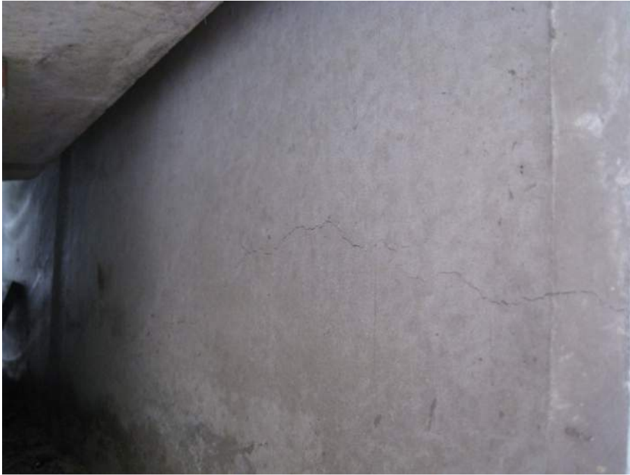
P3 East Wall Cracking
