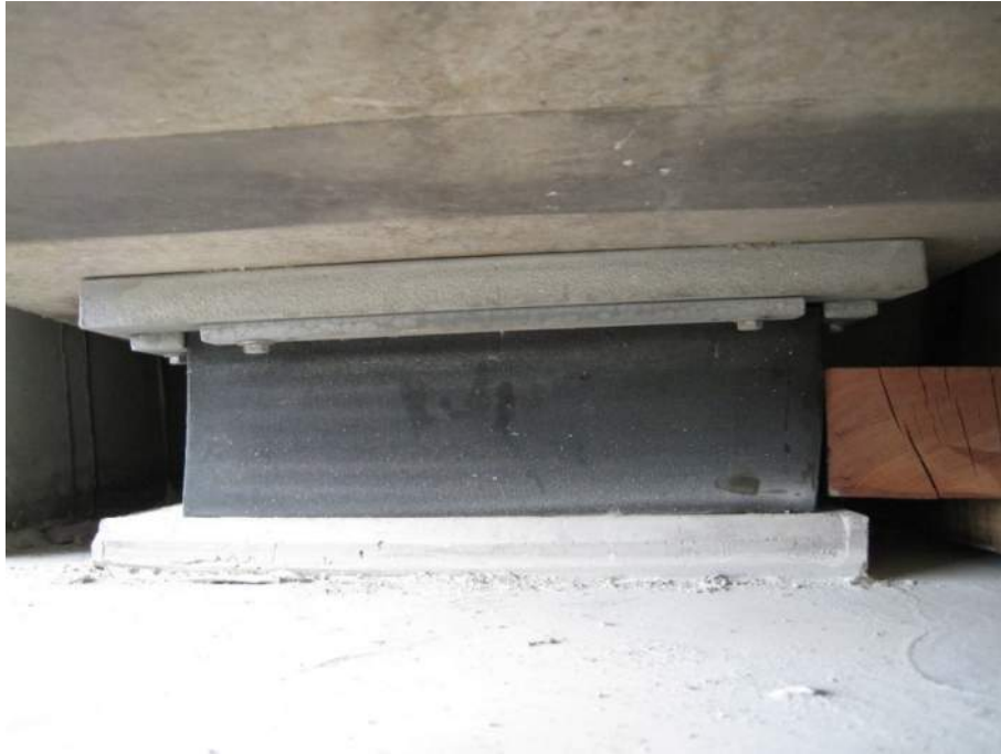
Abutment A Bearing Elevation
