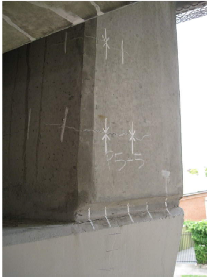
P5 East Wall Cracking
