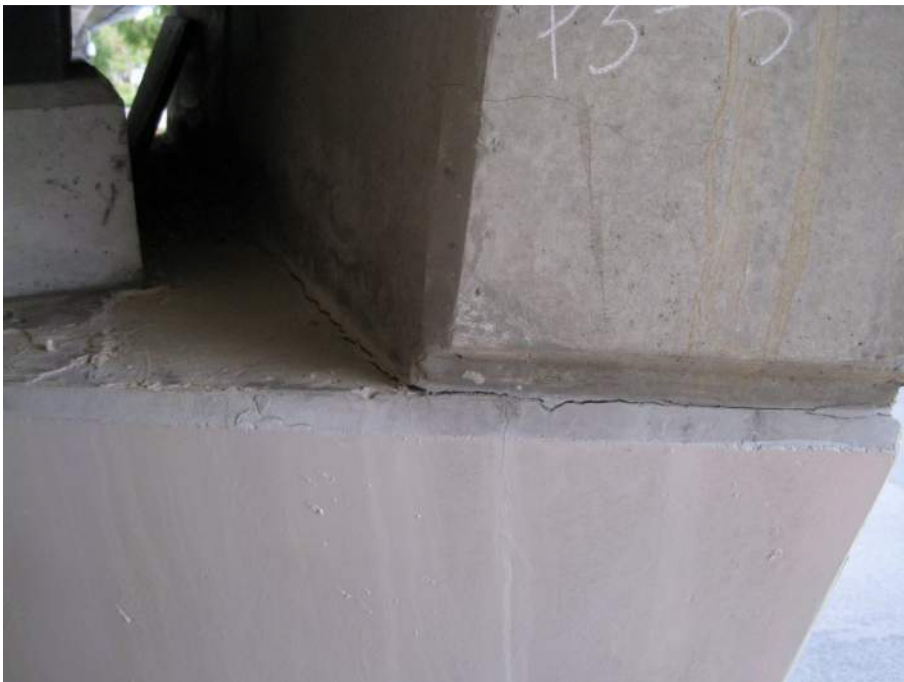
P3 East Wall Cracking
