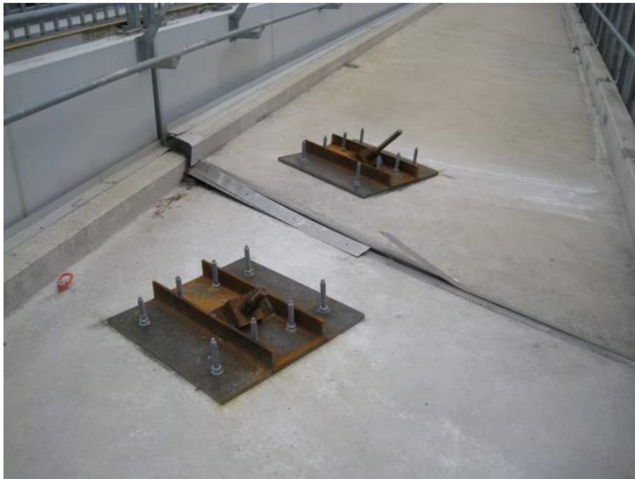
Temporary Tie Anchors Typical
