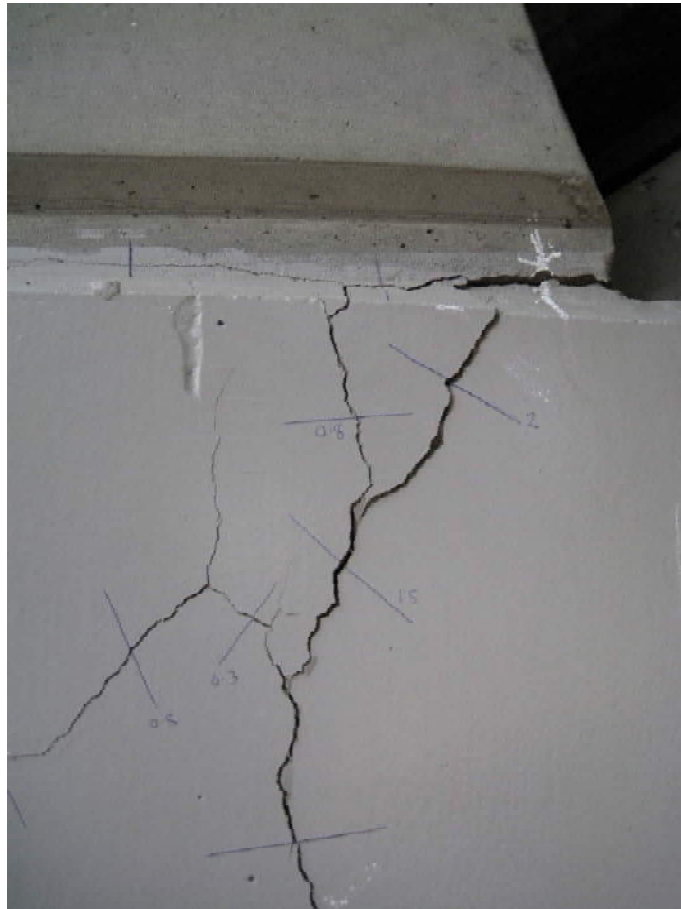
P4 West Wall Cracking
