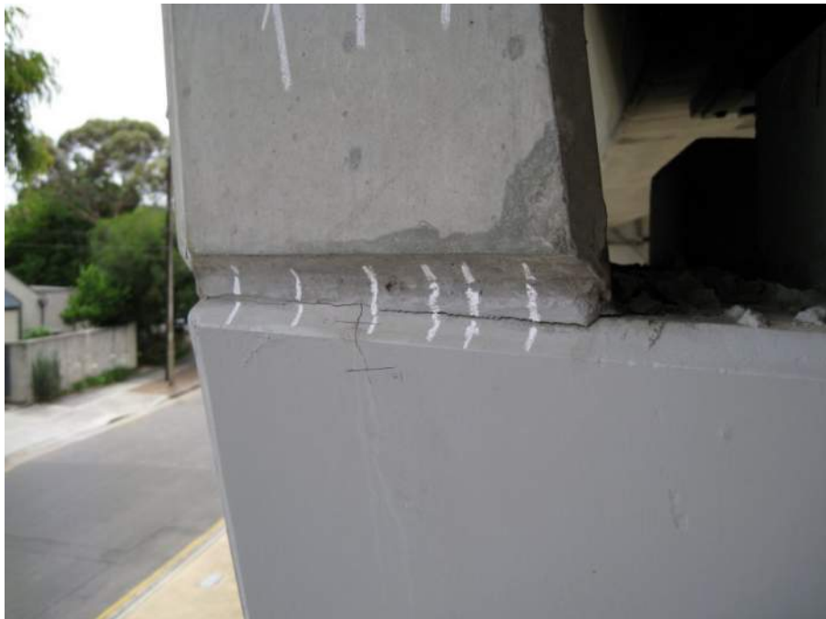
P5 West Wall Cracking
