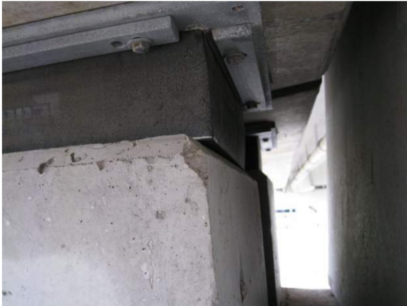
P7 West Bearing Displacement
