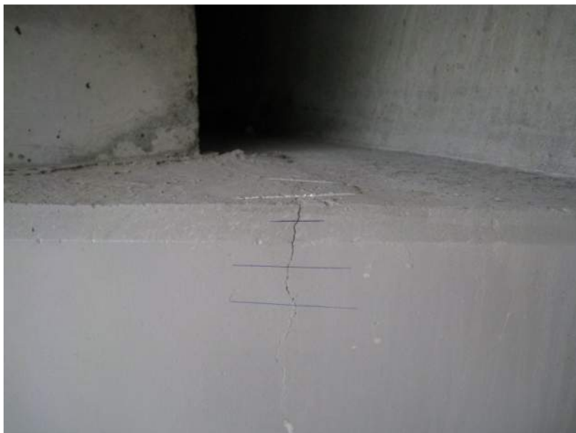
P5 West Headstock Cracks
