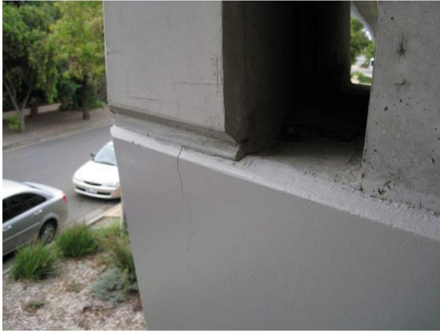
P7 West Wall Cracking
