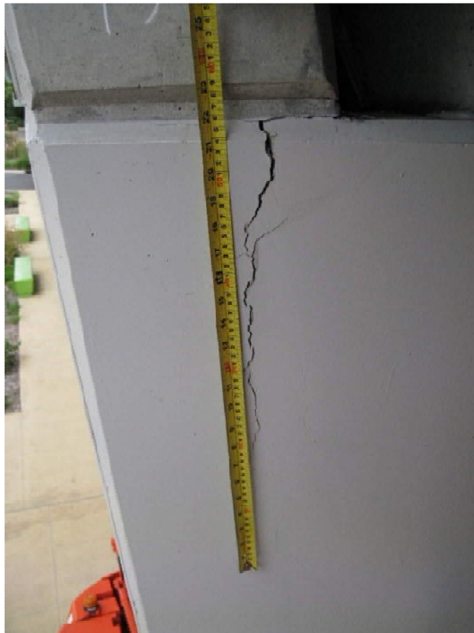
P3 West Wall Cracking
