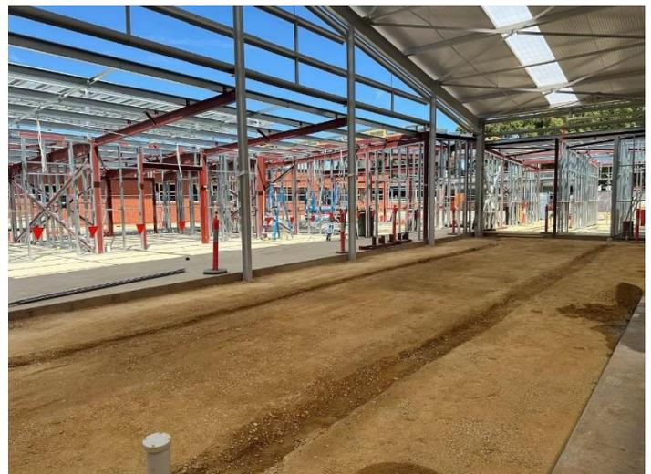
Image: concrete slabs and structural steel installation
