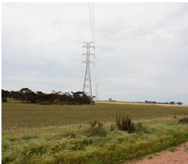
Figure 15 A high voltage electrical easement seen from Hoffman Road (Source: AECOM)
