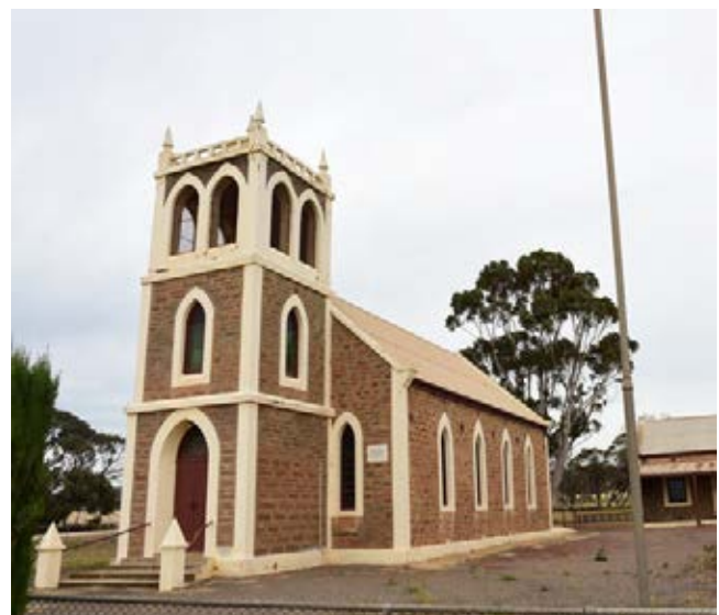
Figure 11 Summerfield Lutheran Church Group (Source: AECOM)
