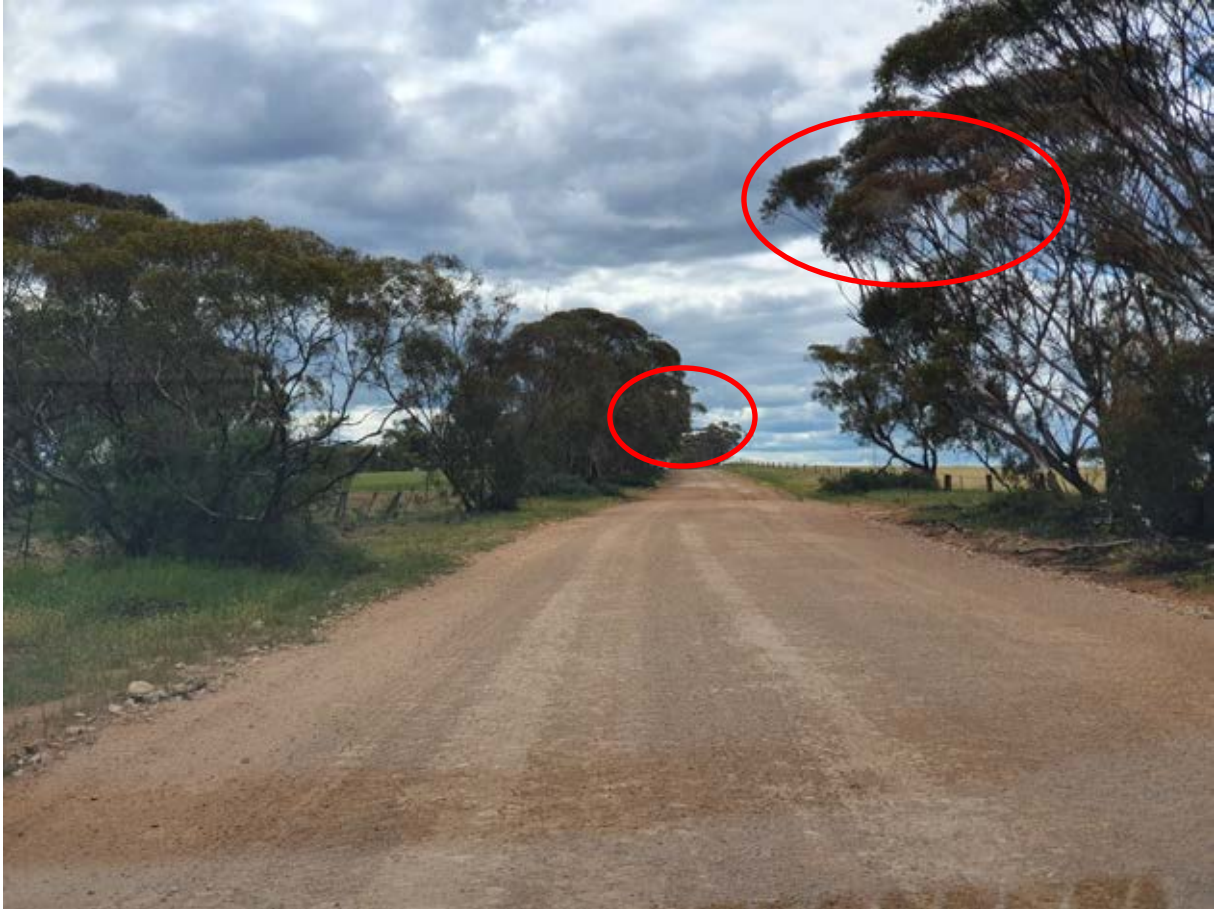
Figure 14 Overhanging vegetation Hoffman Road
