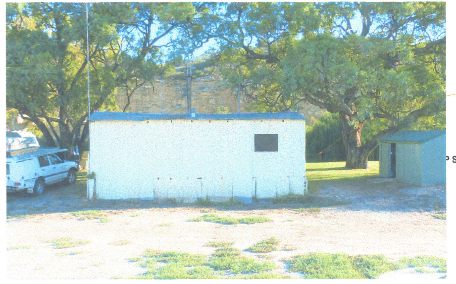
VIEW OF EXISTING SITE
