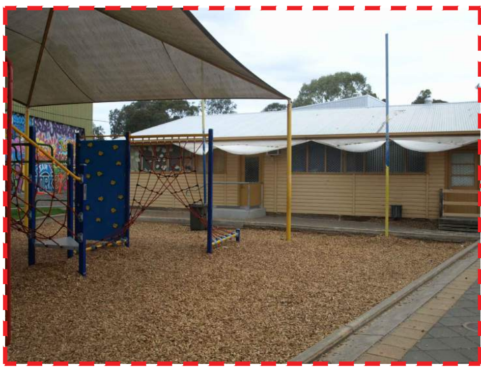
7 - DEMOLISH EXISTING COMMUNITY TRANSPORTABLE BUILDING
