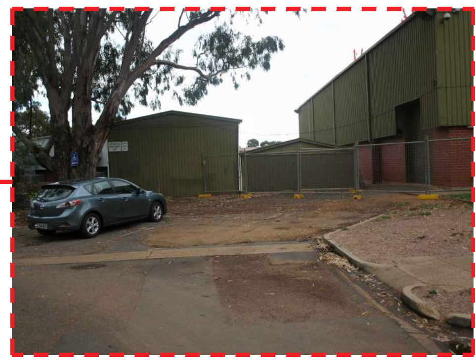
SH 3 & SH6 - DEMOLITION EXISTING COLORBOND SHEDS
