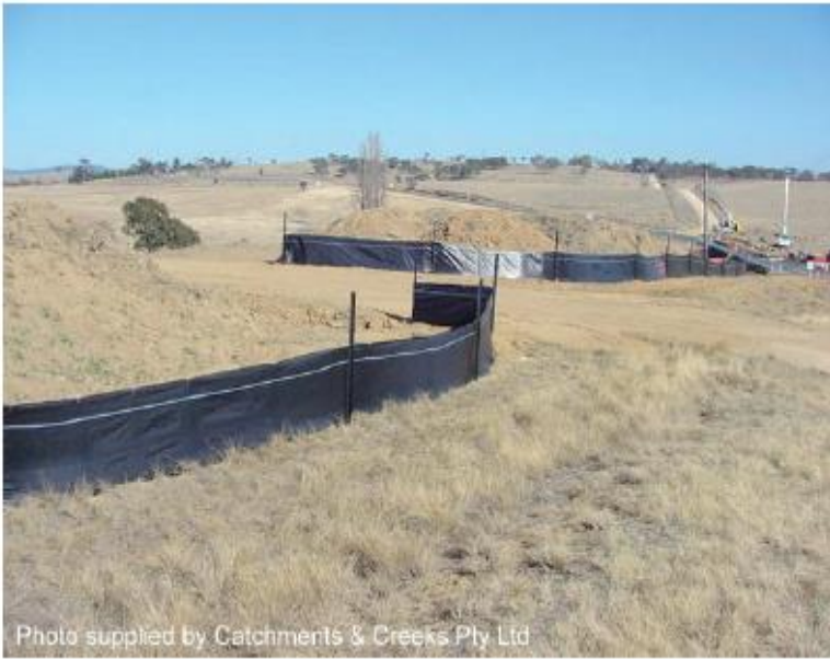
Figure 5 Whoa- Boy Erosion Control Measure – Roads
