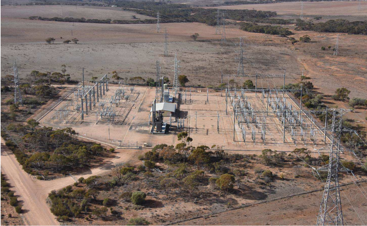
Figure 4-4 Robertstown Substation (current - view looking south east)
