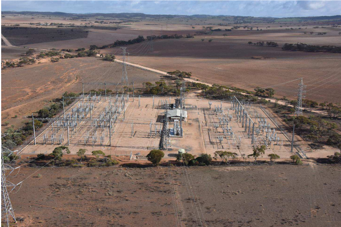
Figure 4-3 Robertstown Substation (current - view looking north)
