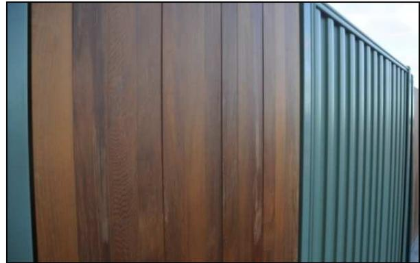
*It is important that timber fences do not have any gaps or cracks for the noise to pass through*
