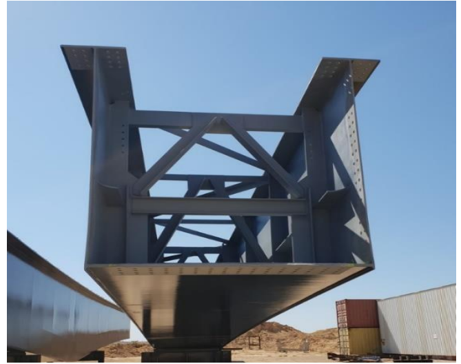
Example of a bridge girder
