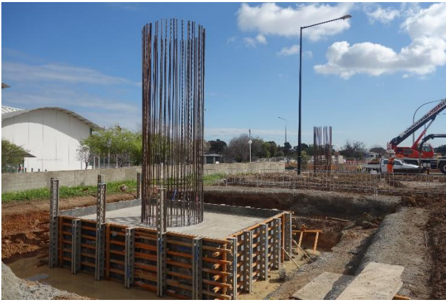
Flinders Link Project pile cap and commencement of pier column
