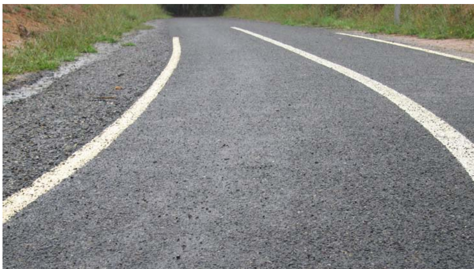
Figure 3.1 Spray sealed bikeway
