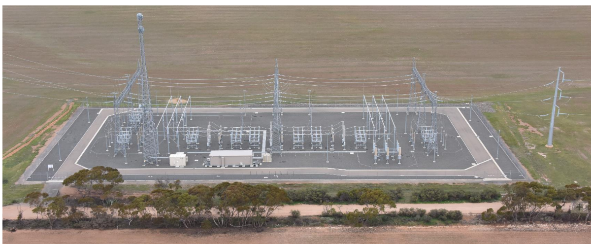
Fig 1.4 Example switchyard yard (North - South)
