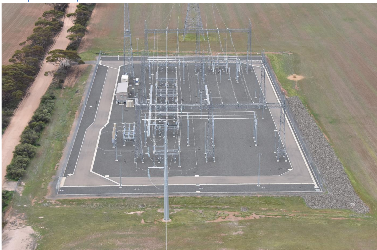
Fig 1.3 Example switchyard yard foot print circa 150m x 80 metres (East - West)
