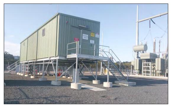
Figure 4-6: Example of a Typical Switch Room
