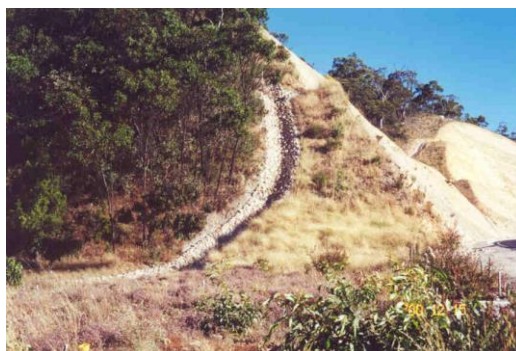
Rock lined drain. Adelaide/Crafers project
