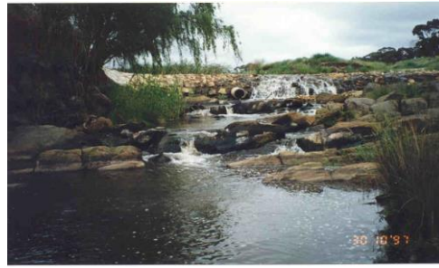
Scour treatment incorporated a fish ladder for native fish.
