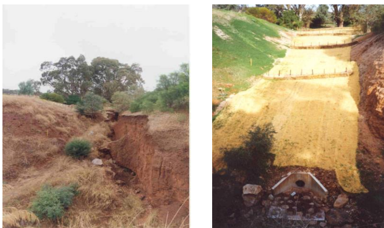
Assess erodibility of soils to prevent scour problems from occurring Cobbler Creek Scour – before and after remedial works
