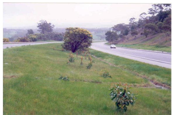
Modified Grass Swale with low-flow drain on South-Eastern Freeway, Stirling
