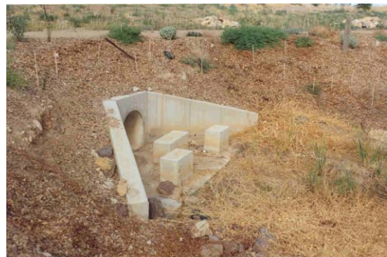
Velocity dissipater on culvert, Field River, Southern Expressway
