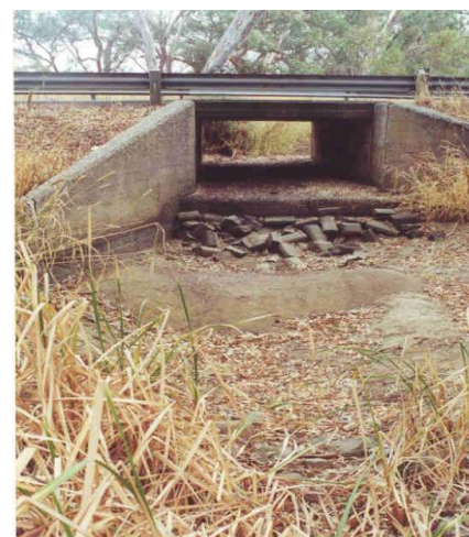
A drop between the culvert and the stream bed can restrict the movement of fish. Brookman Rd, Meadows
