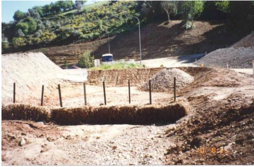
Temporary detention basin. Devils Elbow
