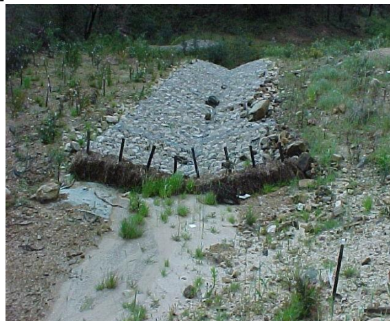
Use a treatment train approach – straw bale, gabion lined channel and sediment basin. Adelaide/ Crafers Project.
