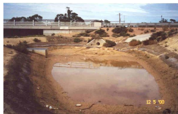
Bridge drainage in a sensitive receiving environment, captured and treated in a detention basin. Blanchetown Bridge, River Murray.
