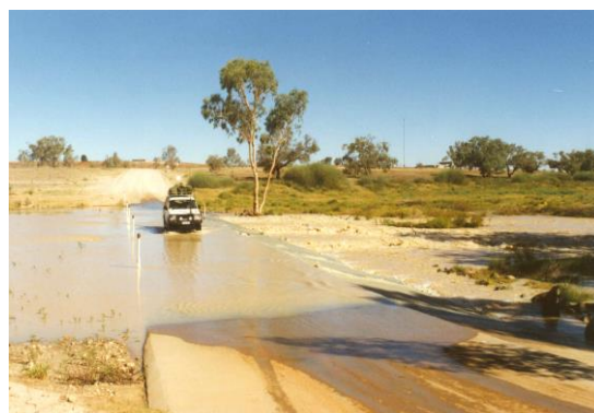
Floodways can create barriers to fish movement. Coopers Creek
