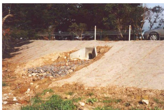
Ensure effective scour protection at drainage outfalls
