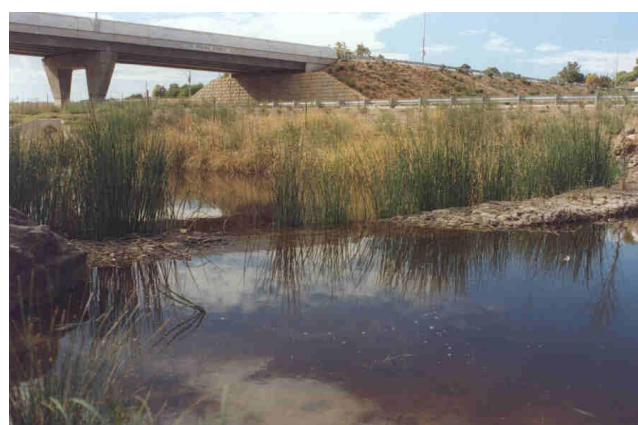
Wetland on Southern Expressway treats road runoff prior to discharge to the Field River
