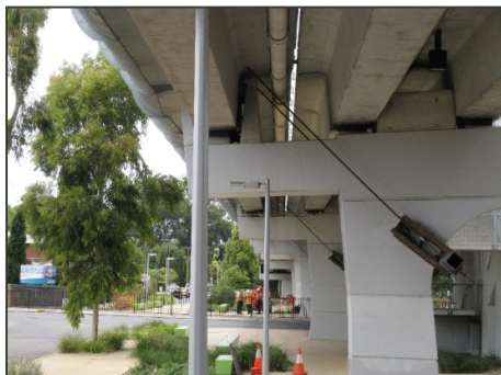
Figure 2 Temporary stabilising tiebacks
