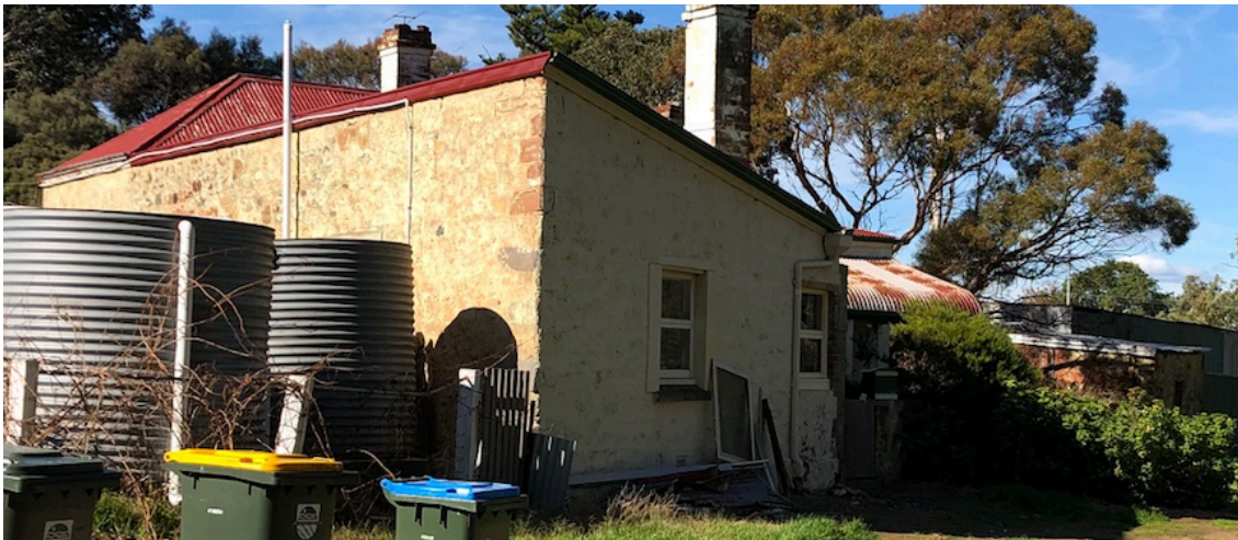
Figure 8. Local building form, Alfred Place, Strathablyn.
