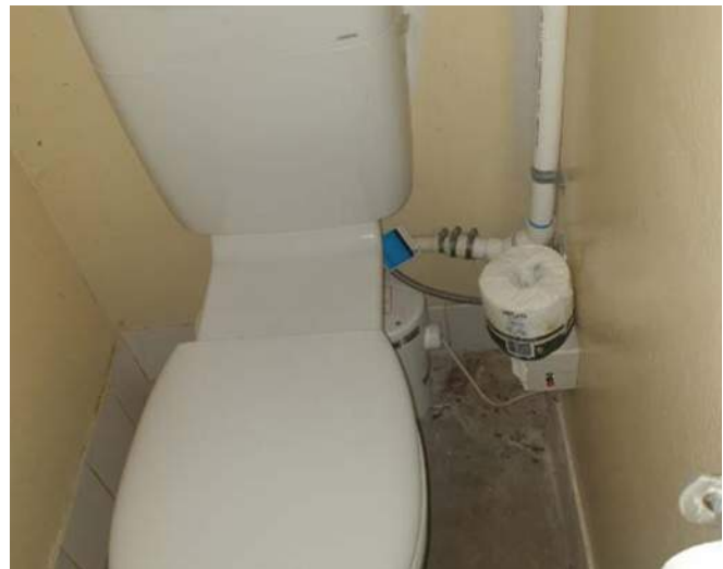
Image 06: Lifting Station behind each WC's
