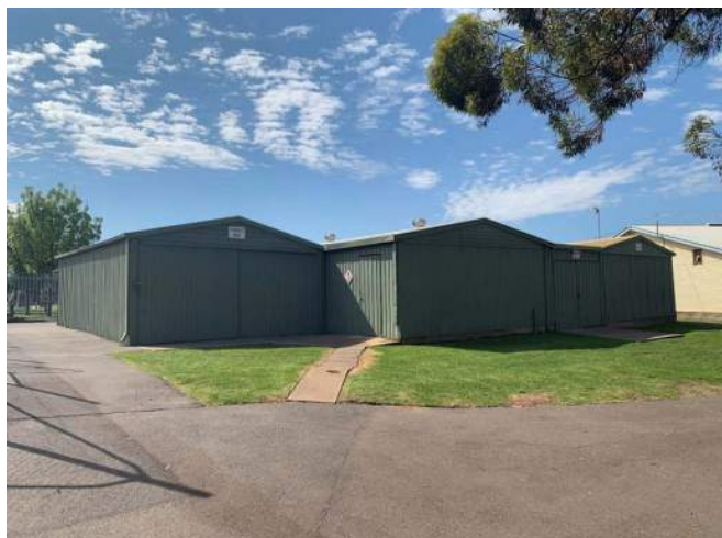
Image 10: Existing sheds, L-R: SH3, SH1, SH6, SH2. Storm water discharges directly to adjacent pavement or grassed area.
