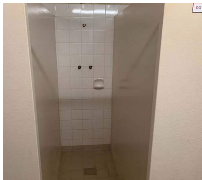
Image 11: Building 4 area considered for refurbishment. Taps removed and drains sealed previously due to failure of pipework under.
