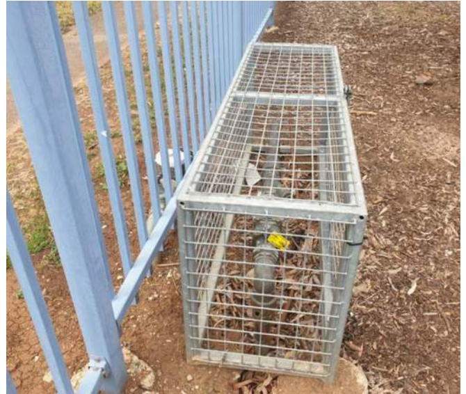
Image 02: Potable Water Meter on Brunel Drive
