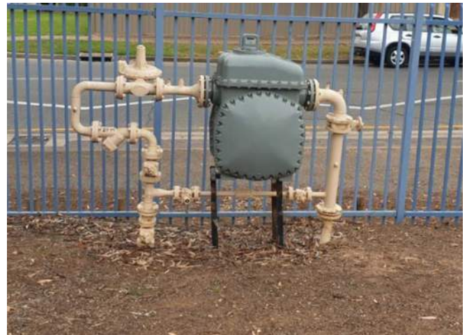
Image 03: Gas Meter on Brunel Drive
