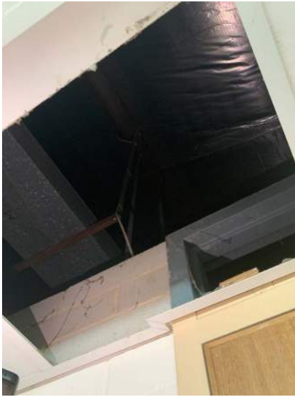
Image 12: Building 4 ceiling space. Walls and ceilings do not comply with current seismic requirements
