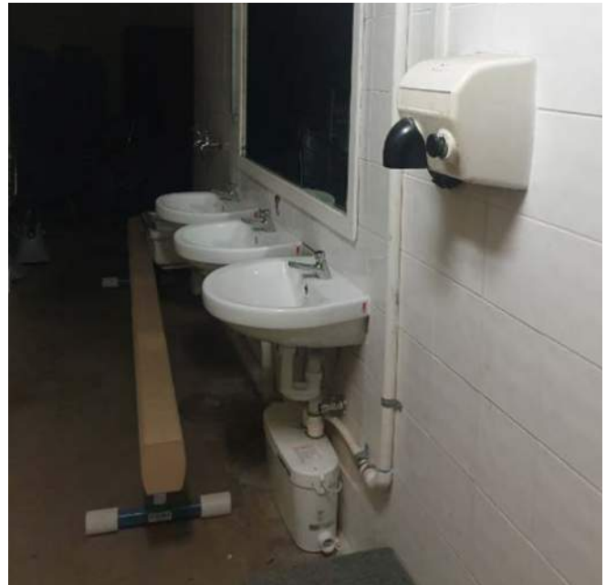
Image 05: Lifting Station
