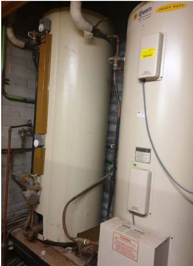
Image 07: Gas hot water system
