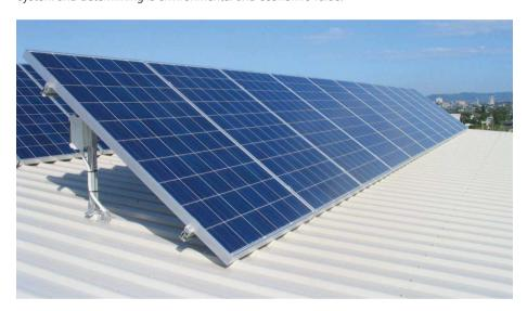
Figure 2.10.1: Roof mounted solar photovoltaic (PV) array
