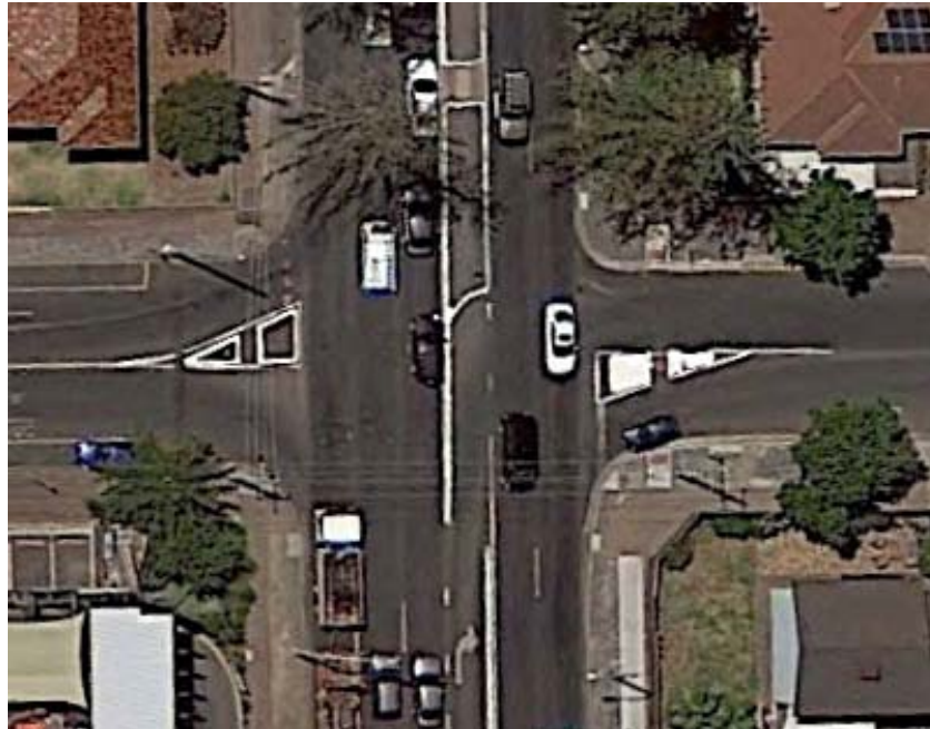
Figure 6-7: Completed Brighton Road / Augusta Street Improvements
