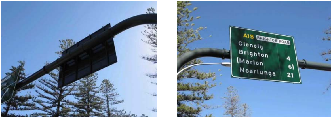
Figure 2-5: Gantry with Advance Directional signage on Brighton Road
