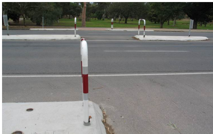
Figure 11.1 Pedestrian/Cyclist Holding Rail
