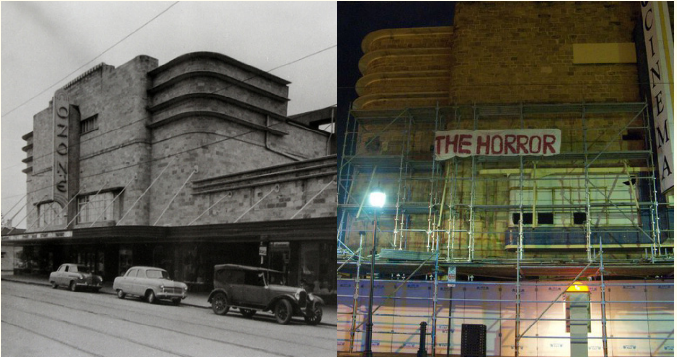
Residents are rightfully horrified by the demolition of local heritage icons.
