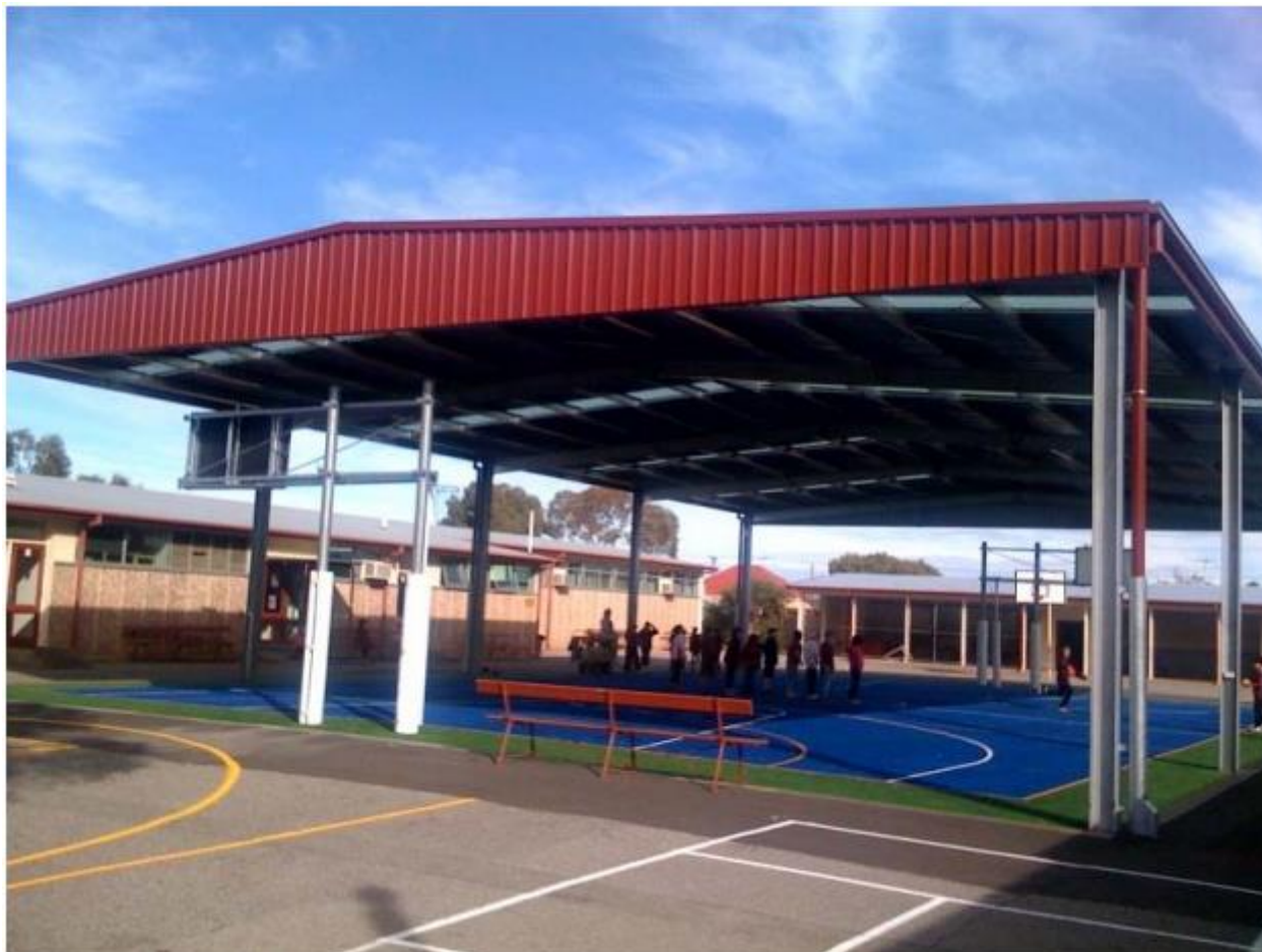
Figure 1. This COLA is located at Murray Bridge South Primary School and was completed in May 2010
