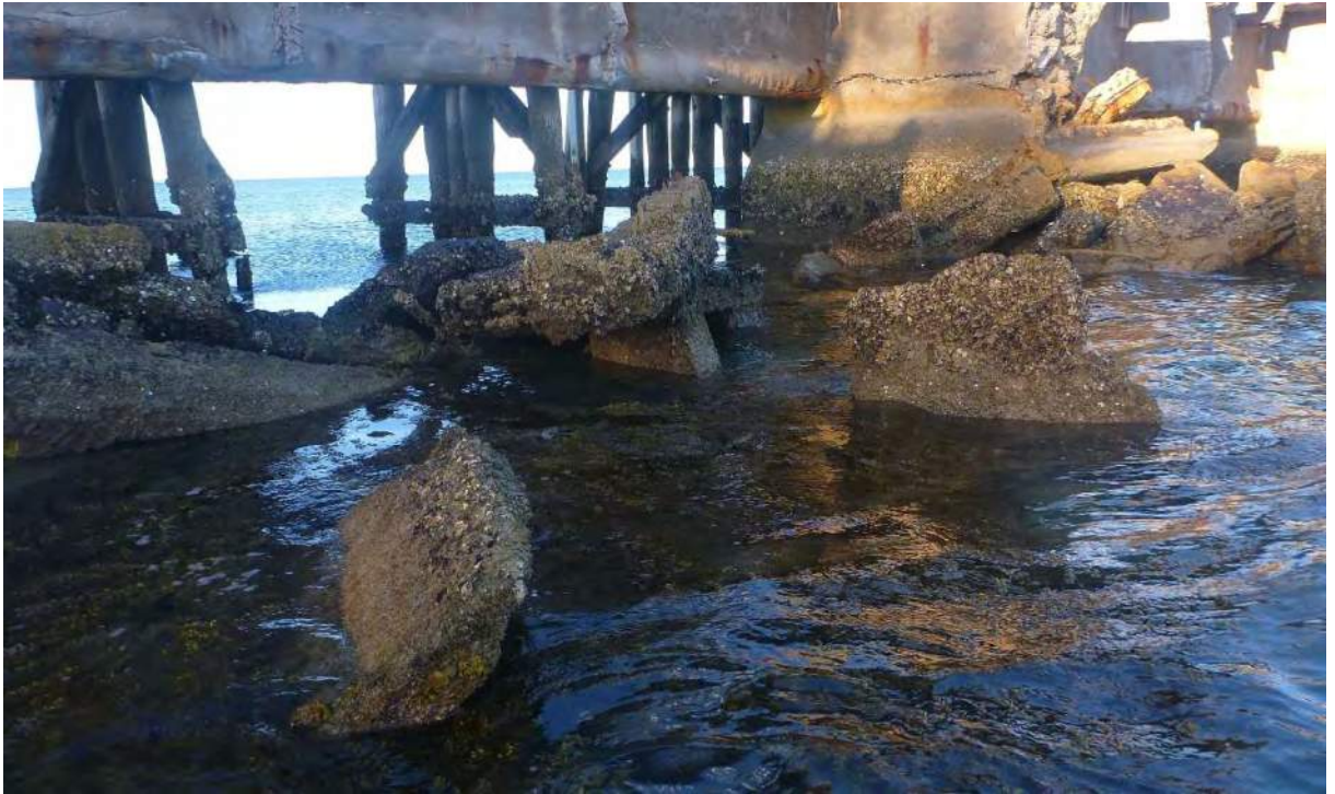
Figure 5-2 Artificial reef structure formed from collapsed sections of the original concrete jetty
