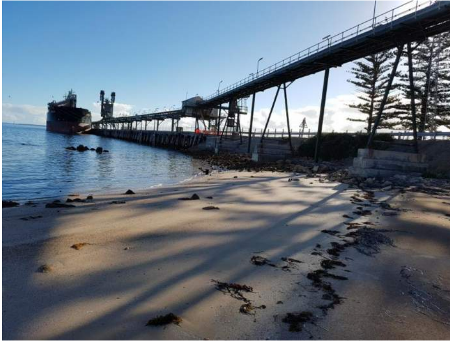
Figure 5: Port Thevenard Jetty groyne
