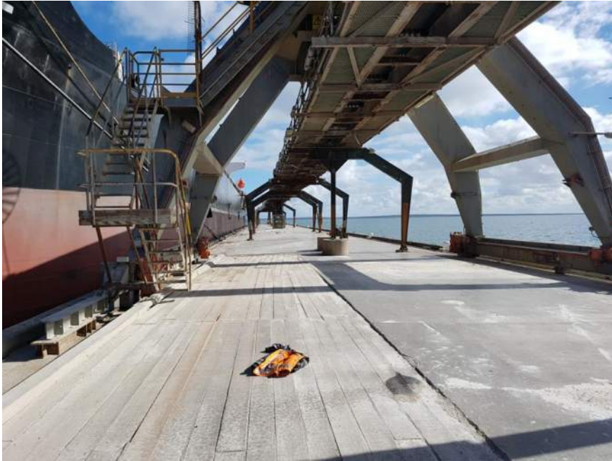
Figure 4: Port Thevenard Jetty Conveyer
