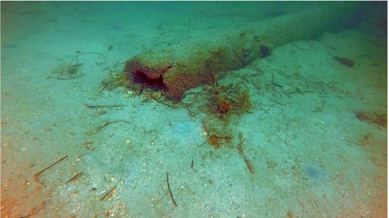
Figure B-5 Pipeline structure with seagrass wrack on rubble substrate
