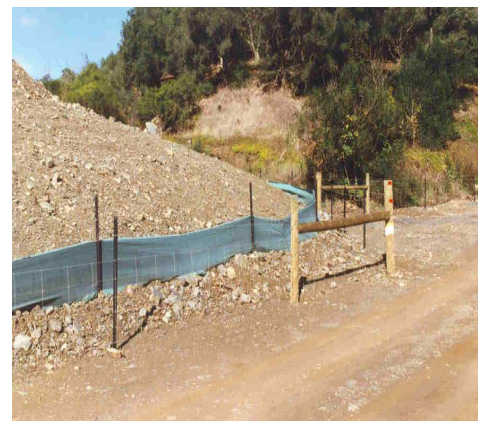
Sediment fence located around a stockpile.
