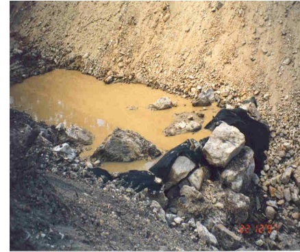
Use site materials to create sediment traps
