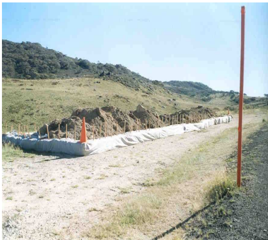
Sediment fence around stockpile - constructed from hay bales and posts.
