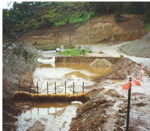
Dry sediment detention basin Adelaide – Crafers project
