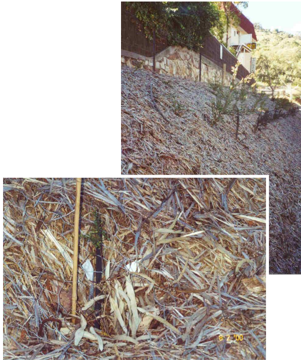
Woodchip mulch secured with mesh is suitable for steep slopes Adelaide - Crafers Project
