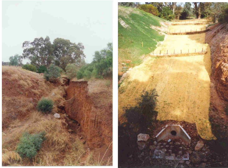
Erosion control matting on severe scour – Cobblers Creek (before and after)
