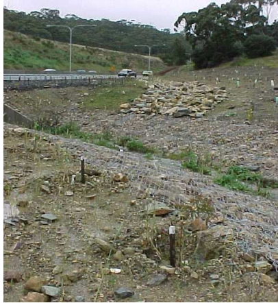
Rock and Gabion stabilisation Adelaide – Crafers Project
