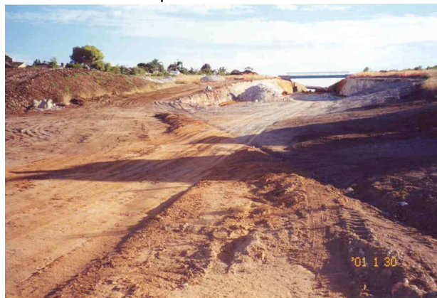
Temporary catch drain
