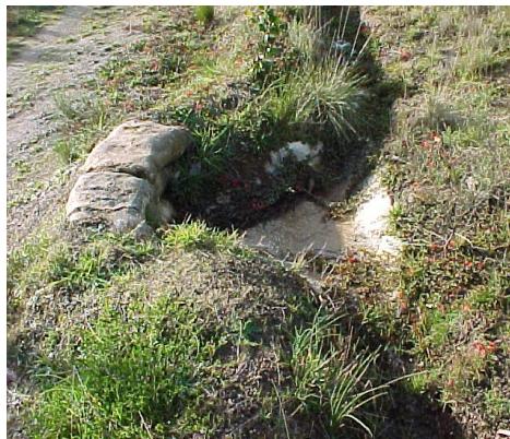
Stabilisation using concrete bags
