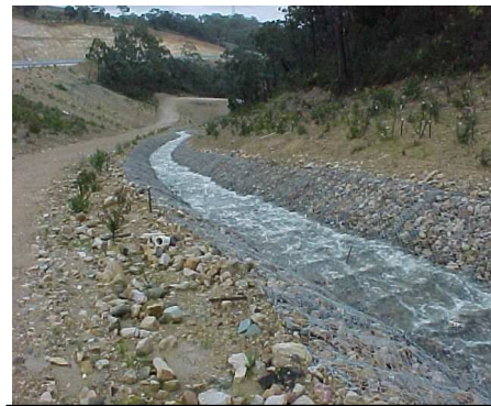
Gabion stabilised drainage line Adelaide – Crafers Project
