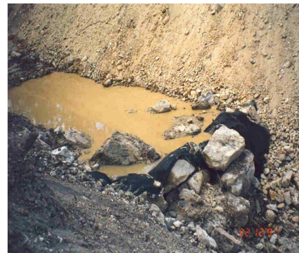
Use site materials to create check dams and minor sediment traps
