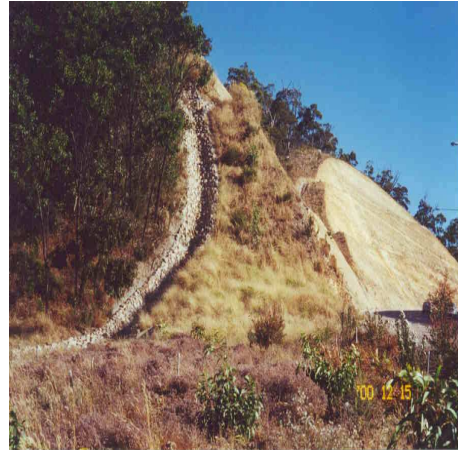
Rock and cement stabilised catch drain outflow Adelaide – Crafers Project
