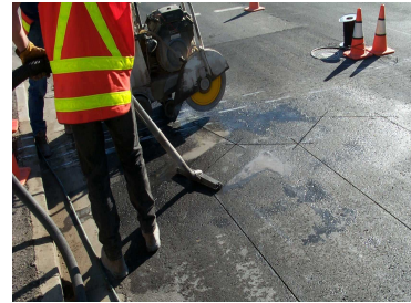
Wet Vacuum during bitumen cutting to reduce the risk of runoff entering the stormwater system
