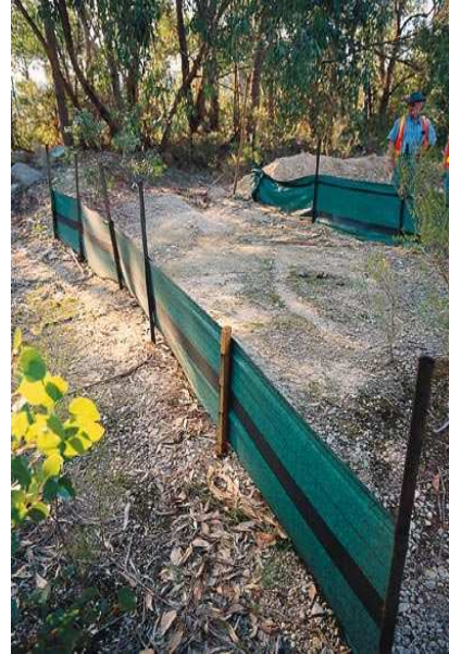
Silt fences used in series
