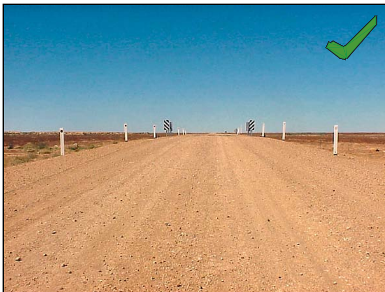
Photo 7 – Correct guide post installation at a grip
