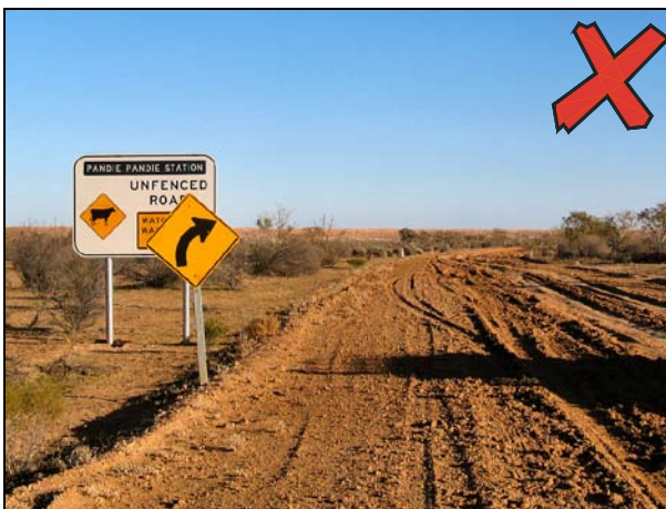
Photo 21 – Signs installed too close
