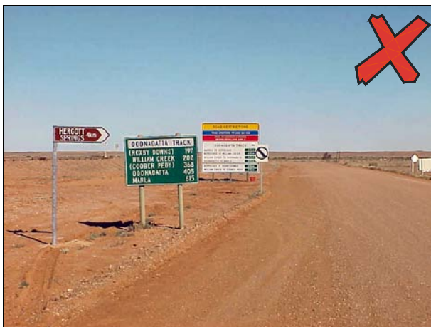
Photo 20 – Signs installed too close and speed de-restriction is not to be used in SA
