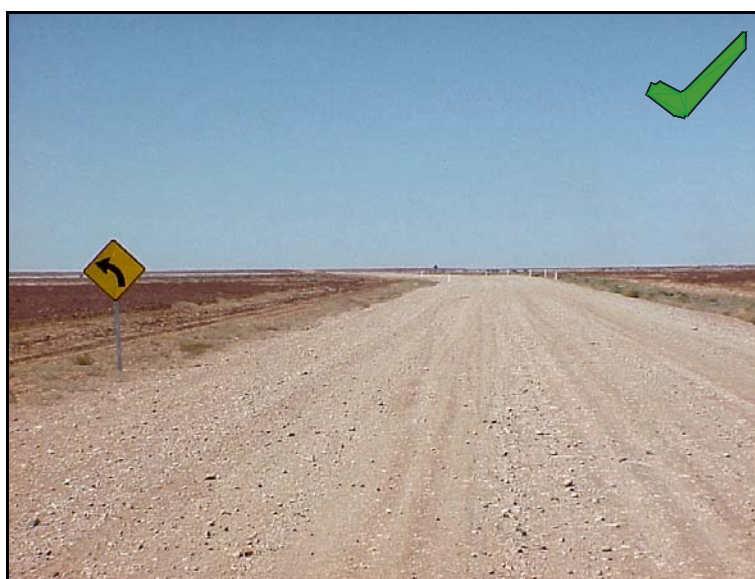
Photo 3 – Correct installation of guide posts and curve sign
