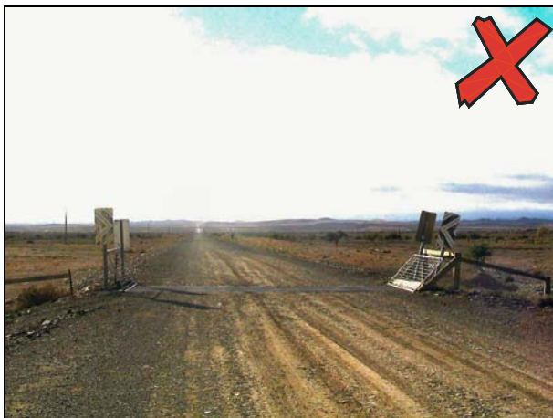
Photo 18 – Wrong hazard markers used and signs in very poor condition
