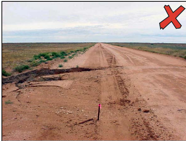
Photo 11 – Inadequate warning for temporary traffic hazards
