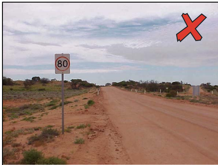
Photo 1 – Incorrect placement of speed sign
