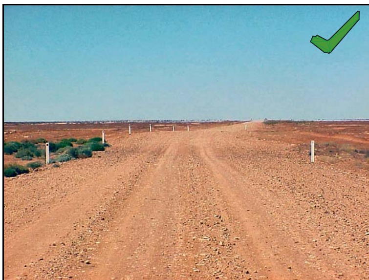
Photo 2 – Correct guide post installation and curve sign not required
