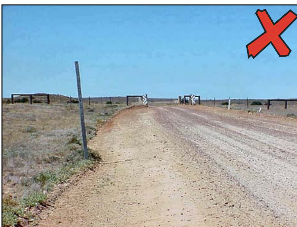
Photo 23 – Sign missing and post installed too close to road edge
