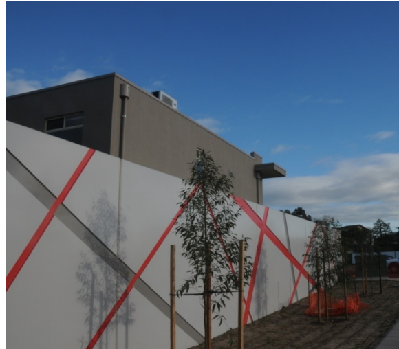
The noise walls at the Gallipoli Underpass were textured and finished to complement the ANZAC theme.
