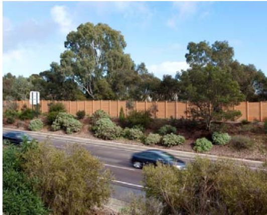
Where space is available, locating a barrier on top of an earth mound can increase its effective height.
