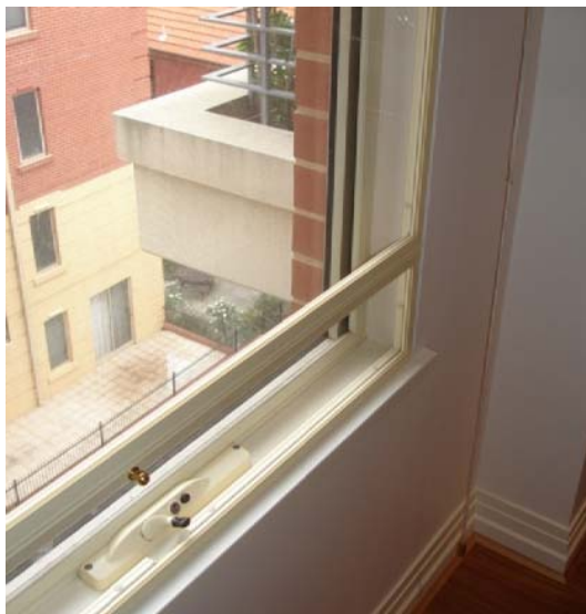
Secondary and double glazing systems are two possible noise mitigation treatments that can produce significant noise reductions if properly installed.
