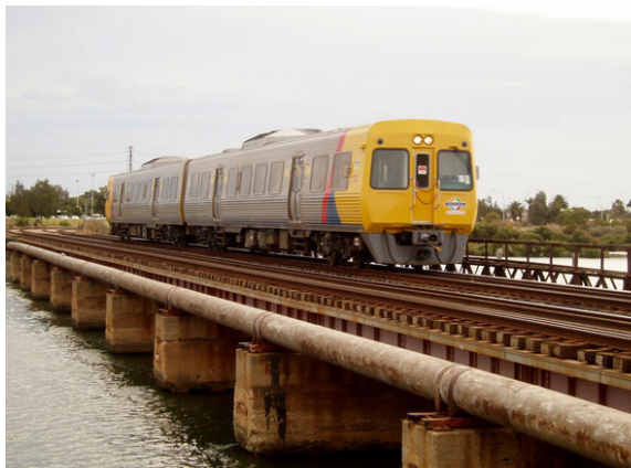
There is no significant difference in noise levels between electric and diesel passenger rail vehicles.
