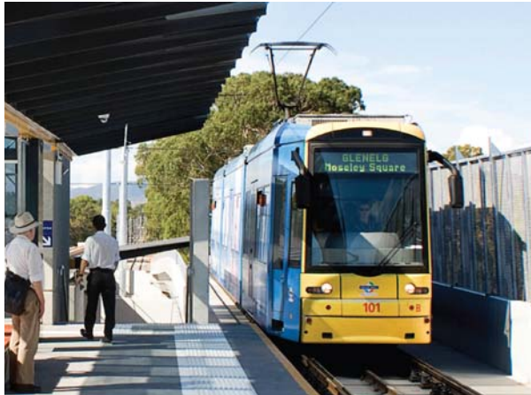
A one metre high concrete barrier on the Glenelg Tram Overpass provided the necessary noise reduction due to the low height of the wheel-rail interface and the raised height of the noise source relative to the receivers.
