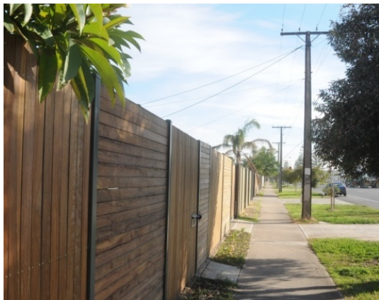
Timber can be used to visually soften roadside barriers but care must be taken to avoid gaps between pieces of timber.
