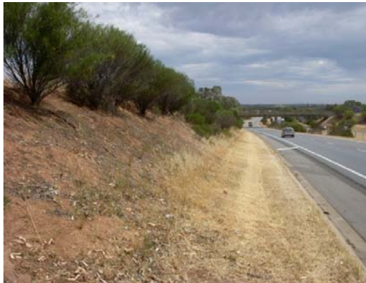
Earth mounds can be designed to be noise barriers with low visual impact.
