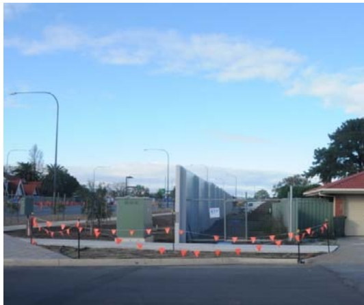
Noise walls must at least break line-of-sight between the road and receiver.
