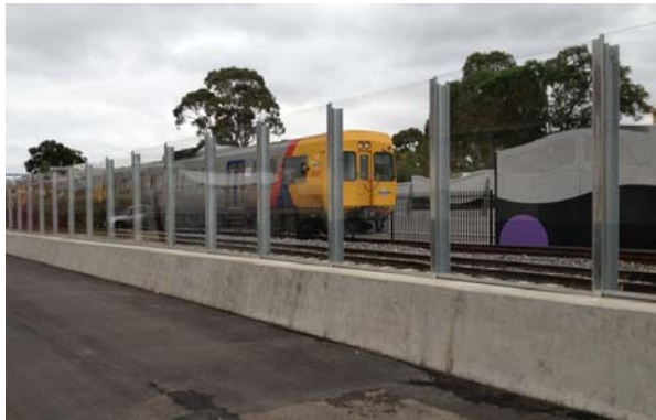
Transparent barriers at Eastlink (Victoria) and Goodwood reduce the overall visual impact and are also useful where views need to be retained.
