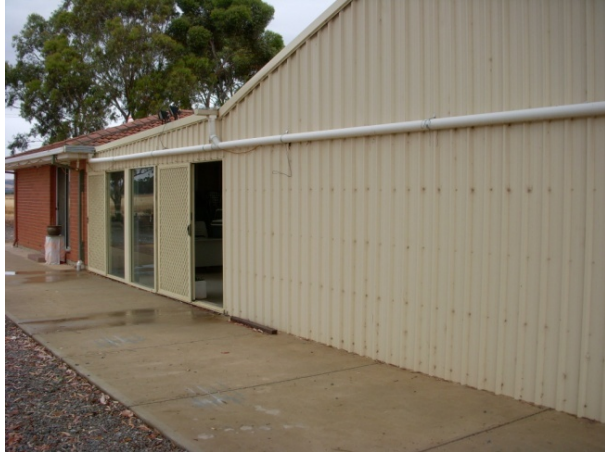
Habitable spaces with lightweight external walls may need wall treatments if they are significantly affected by a transport infrastructure project.
