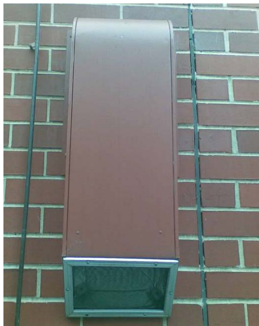
Acoustically treating wall vents, such as this one near the Gallipoli Underpass, is an effective yet unsightly treatment option.
