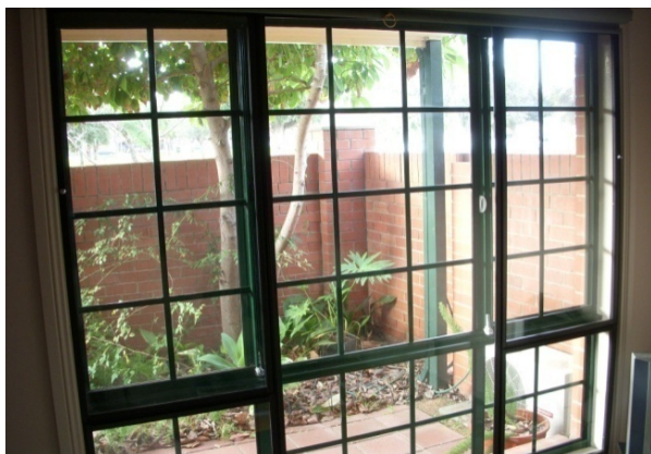
A proprietary acrylic secondary glazing system installed on the internal side of an existing window.
