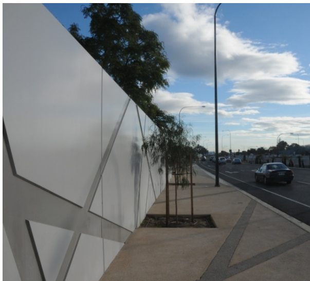
Precast concrete barriers, such as those at the Gallipoli Underpass, are effective noise barriers but are relatively costly.
