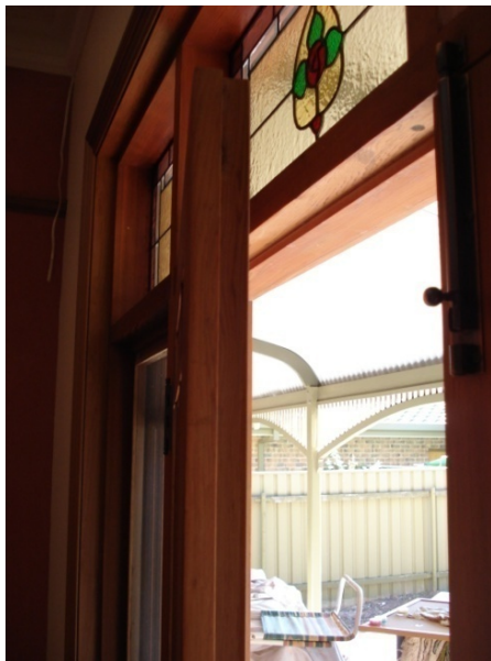
Doors with decorative glass panels in and around them can be difficult to provide acoustic treatments for. If the glazing cannot be replaced with thicker glazing, secondary glazing treatments could be considered.
