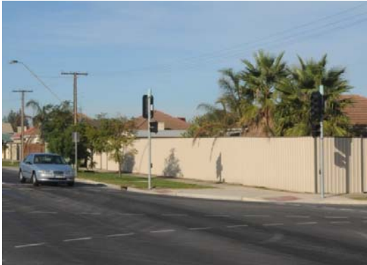
Acoustic fence on a property boundary
