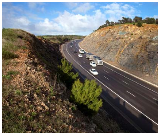
Locating and lowering roads in cuttings will provide natural noise barriers.
