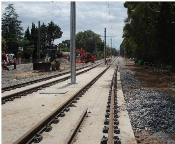
Where a rail track is directly fixed to a concrete base, vibration that generates radiated noise may be a problem. Isolated rail clips, such as these on the Glenelg Tram Overpass, help to reduce the vibration transmitted to the concrete slab.
