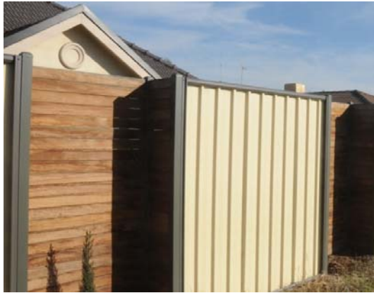
Gaps in barriers, such as in the timber fence shown above, will reduce the noise mitigation achieved.
