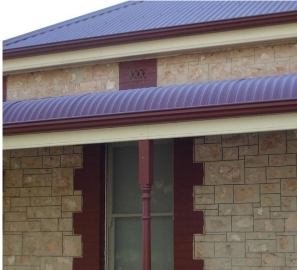
Air vents in a façade requiring property treatment will need to be removed, replaced or acoustically treated.
