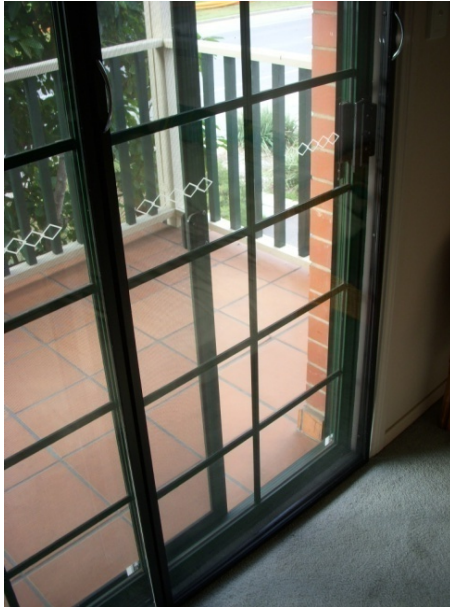
Secondary acrylic glazing installed on magnetic frames on the inside of an existing sliding door.
