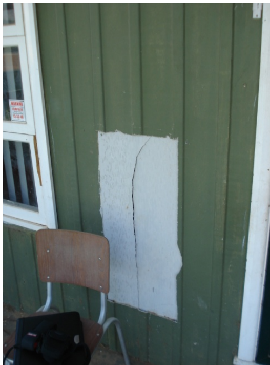
Damage to external walls that could reduce the noise reduction achieved across a facade should be repaired with mastic or with additional wall materials.
