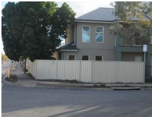
'Colorbond' fence at a property on South Road with a return protecting noise ingress from the side.
