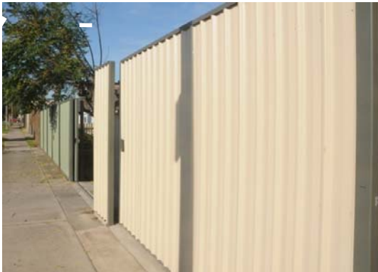
Fences with gates are not normally constructed any higher than 2.1 metres.
