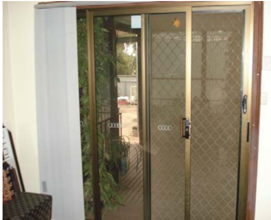
Solid and glazed doors in external building façades represent an acoustic weakness and may require treatment.
