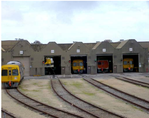
Rail car stabling and maintenance depots can generate significant noise levels, and should be located in non-sensitive areas wherever possible.
