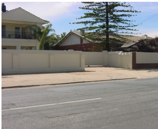
Masonry fence on Portrush Road with a recess to allow a vehicle to enter the driveway.
