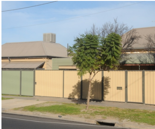
Acoustic fences can provide effective noise mitigation from road traffic, but should break line-of-sight to the road noise sources as a minimum.
