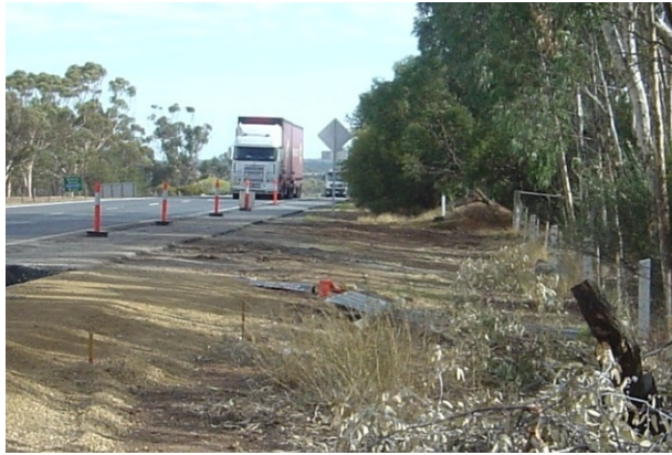
Vegetation adjacent to a road may not reduce noise levels but can block line of sight to the noise source.
