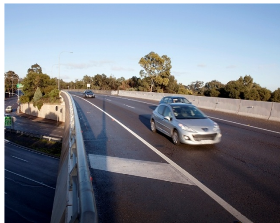
New Jersey style barriers installed on the side of bridges can be effective due to the increased height of the barrier relative to the receiver.
