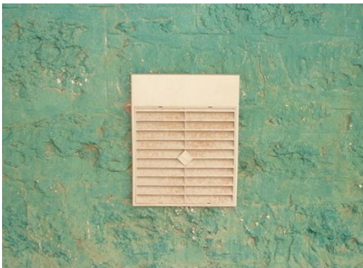
An external view of an acoustically treated air vent. Vents such as this can be used to provide acoustically treated air paths that allow windows to be closed at night time.
