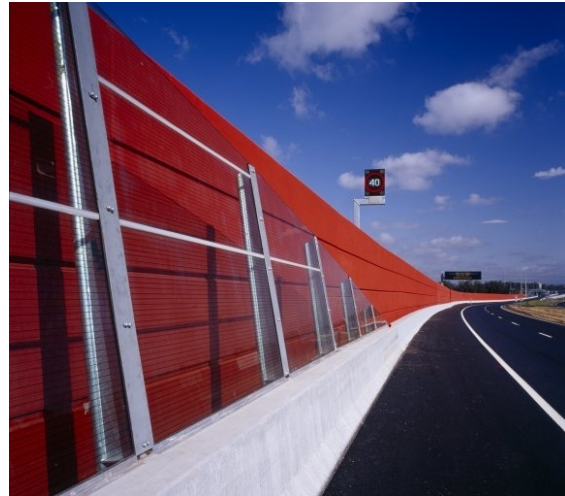
The noise walls on the Westlink M7 in Sydney are angled outwards to enhance the visual effect.
