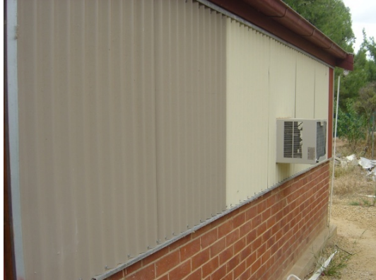
External walls may need to be treated where there are lightweight constructions and openings such as wall-mounted air conditioners.
