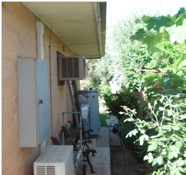
Wall-mounted air conditioners will need to be replaced with an equivalent system in a treated façade.
