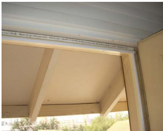
Rubber door seals around the perimeter of a door frame.
