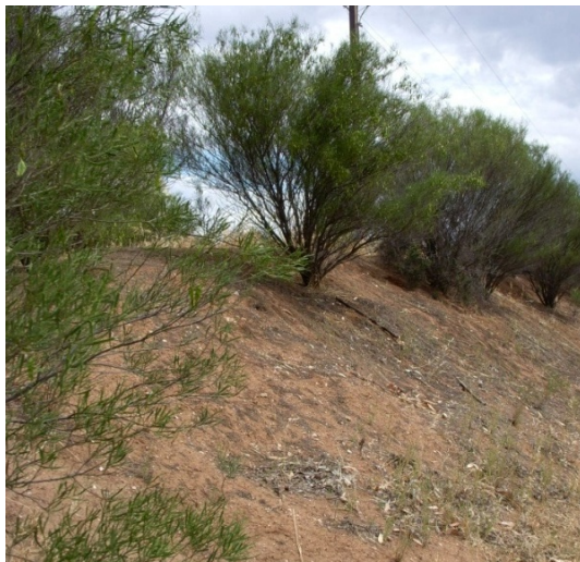
While earth mounds may not require as much maintenance as traditional barriers, it is important to consider well-thought out plantings on the mound so that it does not look bare like the mound shown above.
