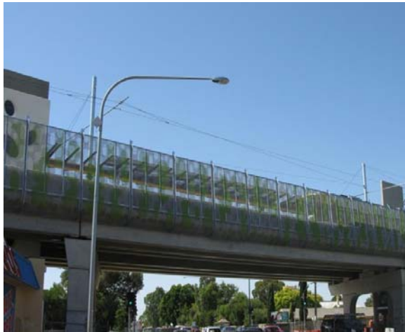
Rail overpasses will result in increased noise levels relative to underpasses.
