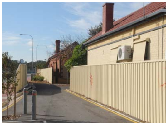
Plain noise barriers with a high degree of public exposure can become targets for graffiti.
