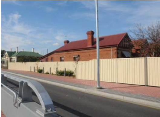
Sheet steel fences are commonly used for acoustic fences less than 2.4 metres high, due to their relatively low cost.
