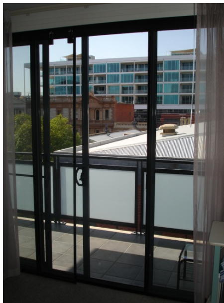
While secondary glazing will mean that two doors need to be opened, it can be a cost effective treatment that does not impact on the appearance of the existing door.
