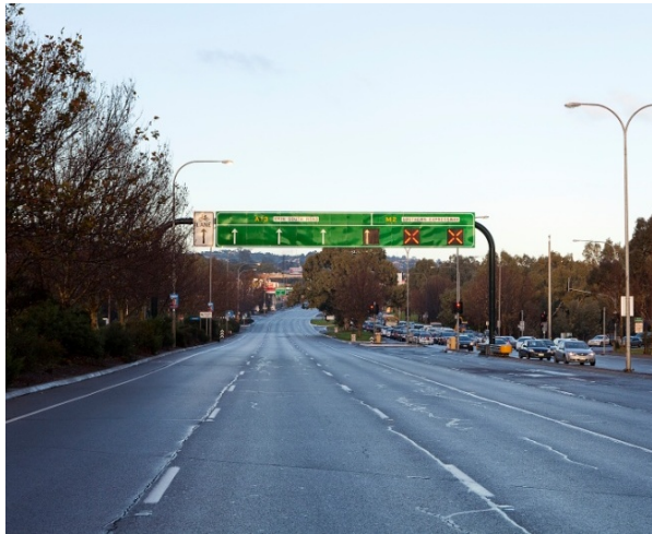
Asphalt road surfaces are less durable than concrete surfaces, but normally produce less noise and can reduce noise mitigation costs.
