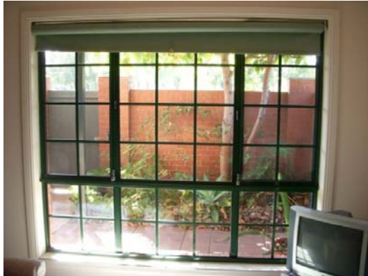
Due to their size and lightweight nature, windows are one of the major noise transmission paths into a room.
