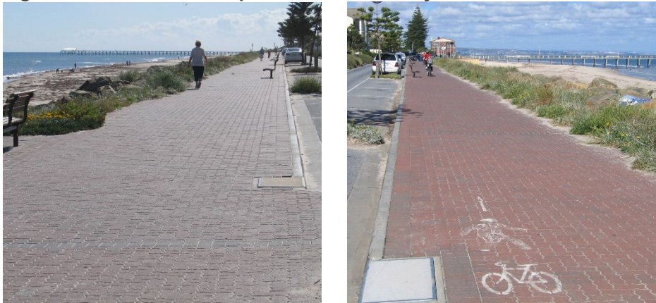
Figure 2-1 Concrete block paver shared bikeway
