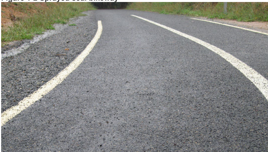
Figure 1-2 Sprayed seal bikeway
